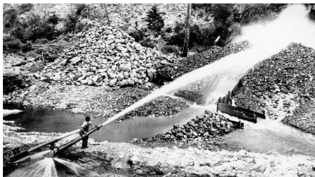
Figure 1-1. Hydraulic miner operates a water cannon.
