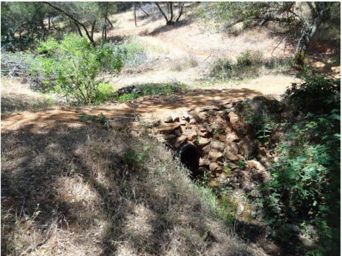
Exhibit 3-19. Typical Stream Crossing using Culvert
