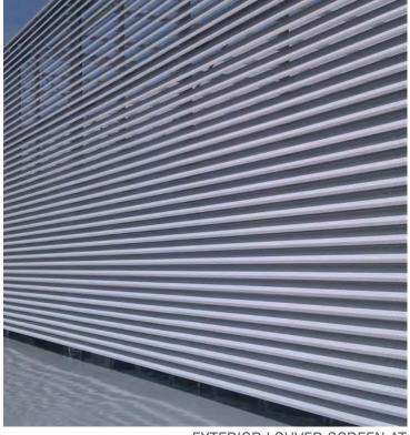
EXTERIOR LOUVER SCREEN AT MECHANICAL EQUIPMENT
