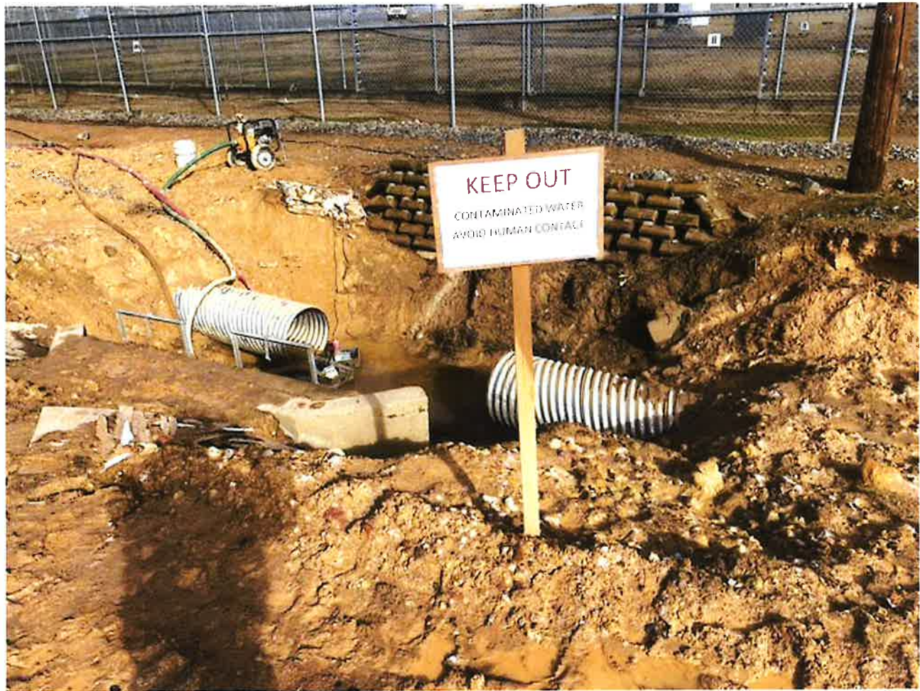
A sign warns of contaminated water. The pumps seen near the pipe are directing the flow from the main outfall back to the Tower 3 cleanout.
