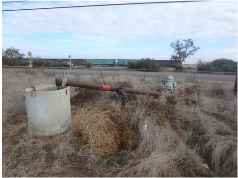
Feature 6: water pump with attached metal pipe extended to a concrete pipe, looking east (Photo P1030037).
