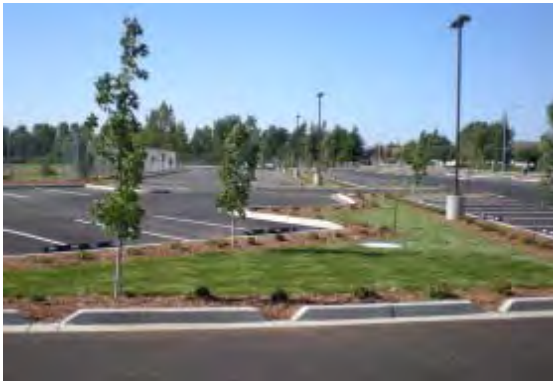
LEFT: Parking lot bioretention in Manteca, CA (San Joaquin Valley Stormwater Quality Partnership) RIGHT: Parking lot bioretention in El Monte, CA (LID Center, LID Manual for Southern California, 2010)
