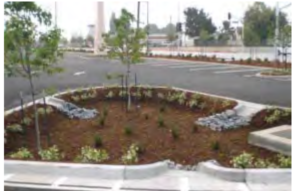
LEFT: Parking lot bioretention in Manteca, CA (San Joaquin Valley Stormwater Quality Partnership) RIGHT: Parking lot bioretention in El Monte, CA (LID Center, LID Manual for Southern California, 2010)
