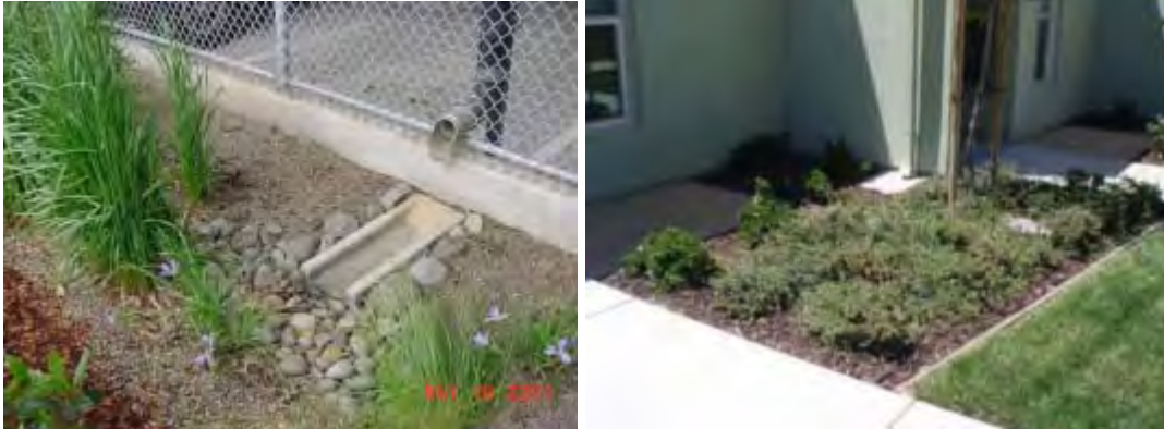
LEFT: Prince George's County, MD (MD Department of Environmental Resources) RIGHT: Downspout disconnection with concrete splash pad.
