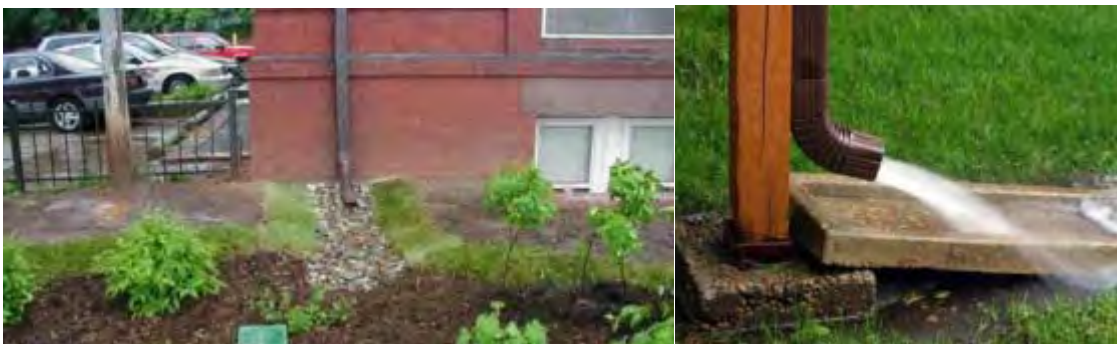
LEFT: Disconnected downspout with rip-rap splash pad. RIGHT: Close-up of disconnected downspout.
