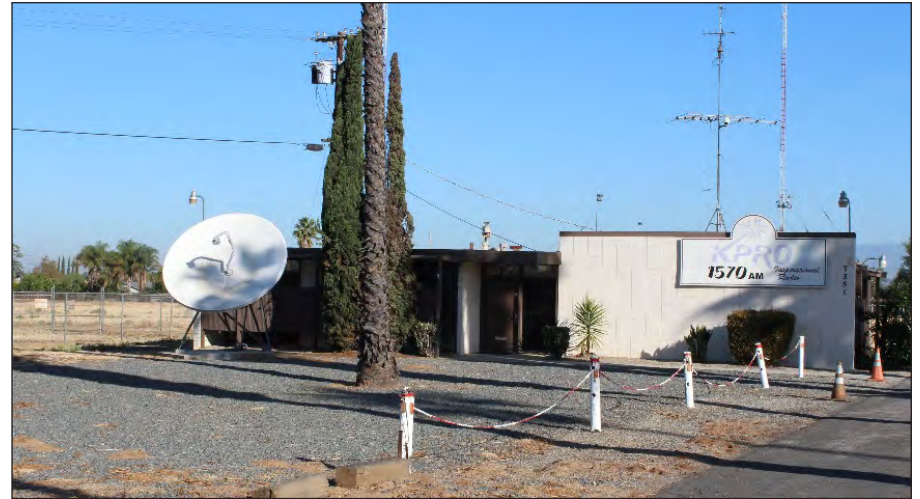
Photograph 2: View of the KPRO broadcasting building, pole-mounted transformers, satellite dishes, antenna, and guyed radio tower structure.
