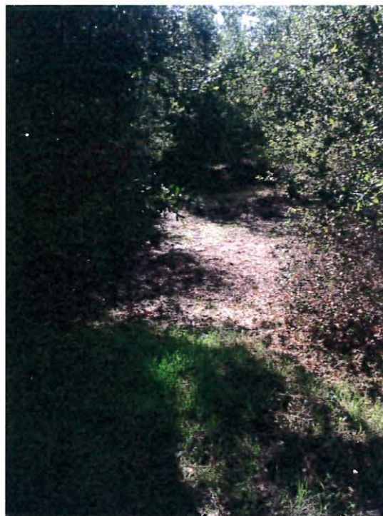
Photograph #2 View of Pipeline Alignment to Freedom Blvd.
