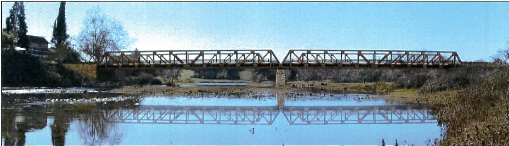
Proposed 2-Span Metal Pony Truss Bridge, looking east.
