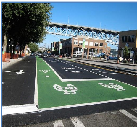
Bike Boxes provide priority to cyclists and safe left-turn movement at traffic signals
