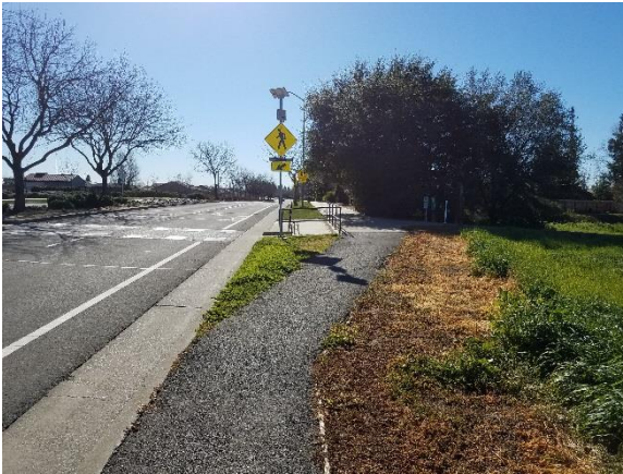
Pedestrian Push Button with Flashing Beacon Warning Sign
