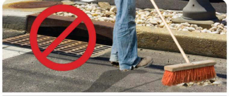
Sweep dry residue or vacuum wet concrete residue and dispose of **properly.** Create a designated washout area for equipment and tools and place away from driveways and storm drains. Dispose of concrete/plaster waste and rinsewater by hauling off to an approved disposal site.
