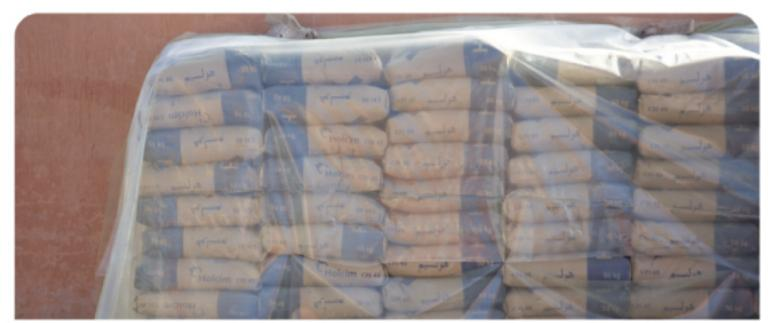
Isolate area and secure bags of cement after they are open. Keep cement, sand and aggregate (wet/dry) and slurries from saw cutting, from flowing into the streets, gutter and storm drains or being blown away. Cover bags of cement in case of rain.
