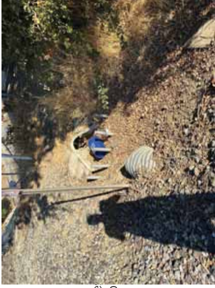
Crosses under railroad track where it discharges to a concrete drop structure
