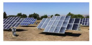
**Typical Dual-Axis Tracking Solar Panels**
