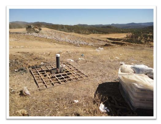
Photo 1. Landfill Gas Extraction Well Installation.
