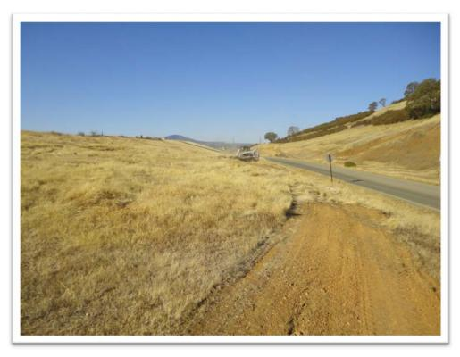
Photo 4. Clearing and Grubbing of Above Grade Header Location.
