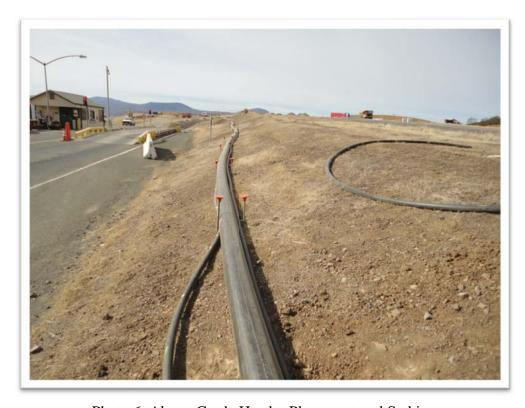
Photo 6. Above Grade Header Placement and Staking.
