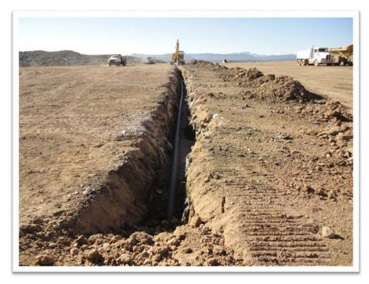
Photo 2. Landfill Gas Horizontal Collector Installation.
