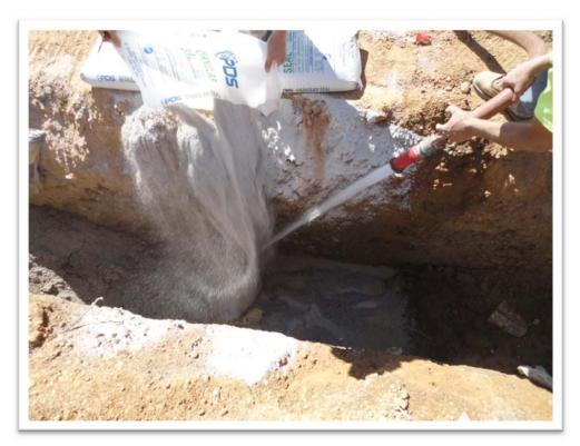
Photo 3. Landfill Gas Horizontal Collector Bentonite Plug Installation.
