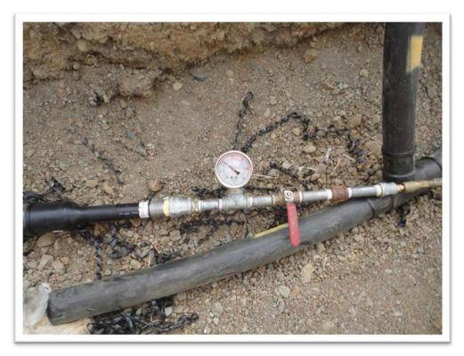
Photo 8. Pressure Testing of Landfill Gas Air Lines and Landfill Gas Header.
