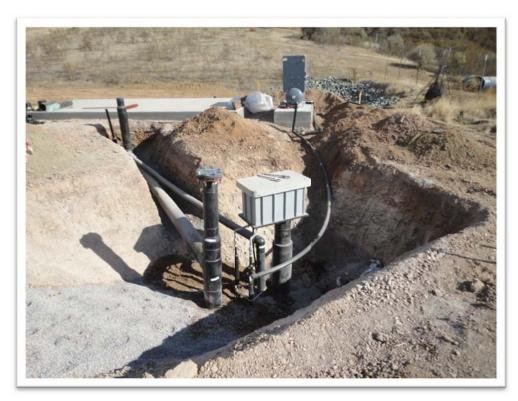
Photo 9. Condensate Trap Installation and Backfill.
