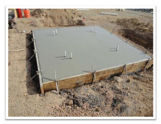
Photo 7. Flare Station Pad Concrete Installation.
