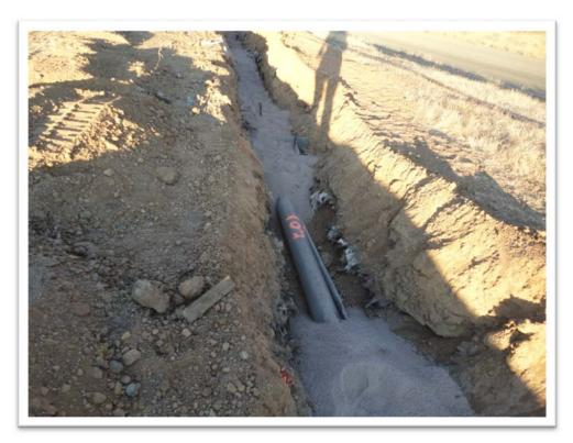
Photo 5. Below Grade Header Placement and Backfill.
