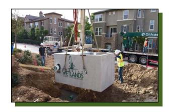
It is the contractor's responsibility to provide suitable lifting equipment to off-load the Modular Wetland unit.
