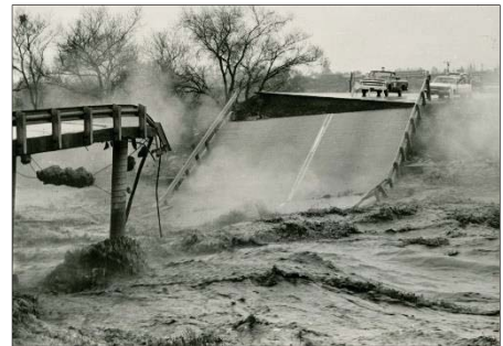
Figure 8-8: Van Buren Bridge collapse during the 1969 Santa Ana River flood (Riverside County Flood Control and Water Conservation District)
