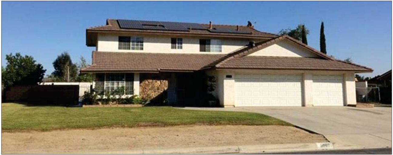
Figure 4-13: Residential roof-mounted photovoltaic solar collectors
