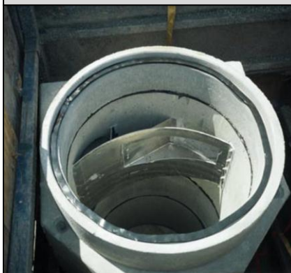
Hydrodynamic Separation Device Source: Contech Stormwater Solution, Inc.
