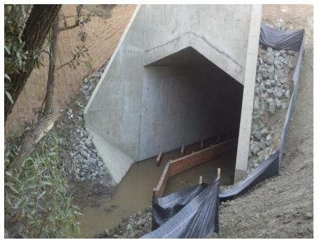
Photograph 3. Headwall of concrete box culvert constructed in 2012.
