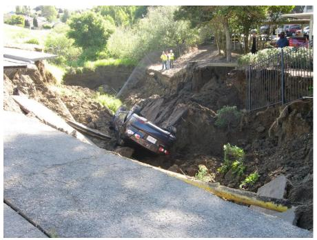
Photograph 1. Via Verdi CMP culvert collapse in April 2010 near the El Portal Drive intersection.
