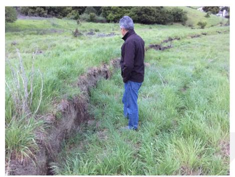
Photograph 10. Landslide scarp along Via Verdi. Photo taken in March 2017.
