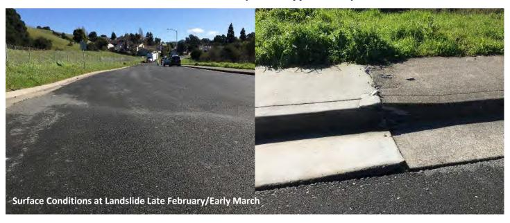
Verdi roadway with the extent of the scarp approximately shown on the **Plate 1**, **Site Plan**. In late February the landslide was observable as undulations/settlement with some cracking in the asphalt pavement and concrete sidewalk as shown in the photos above with
