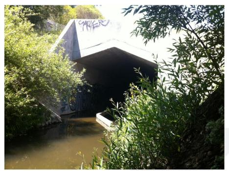
Photograph 8. Existing Via Verdi culvert headwall, location of the proposed culvert tie-in.
