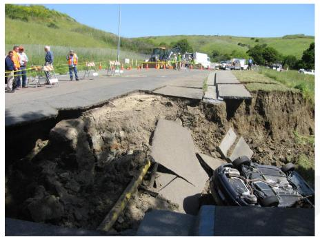
Photograph 2. Via Verdi CMP culvert collapse in April 2010 near the El Portal Drive intersection.
