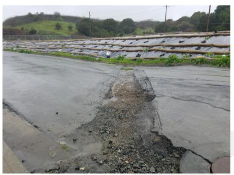
Photograph 16. Uneven condition of the existing Via Verdi roadway. Photo taken in January 2018.
