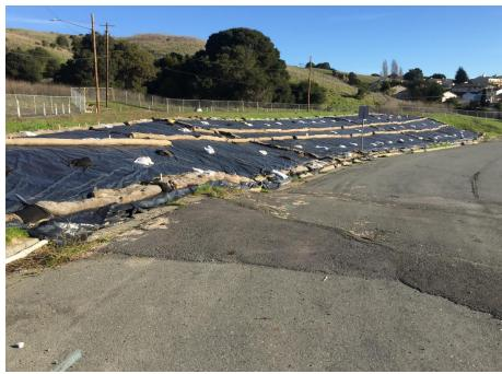
Photograph 15. Detail of existing Via Verdi and landslide conditions. Photo taken in January 2019.
