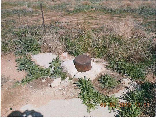
PHOTOGRAPH 4 – Close-up view of the steel riser pipe observed in the northeasterly portion of the concrete foundations area near the east central property boundary. This is estimated to be the location of a capped water well.
