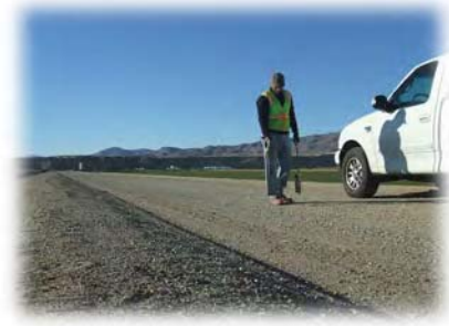
Electromagnetic (EM) utility location (archive photo)
