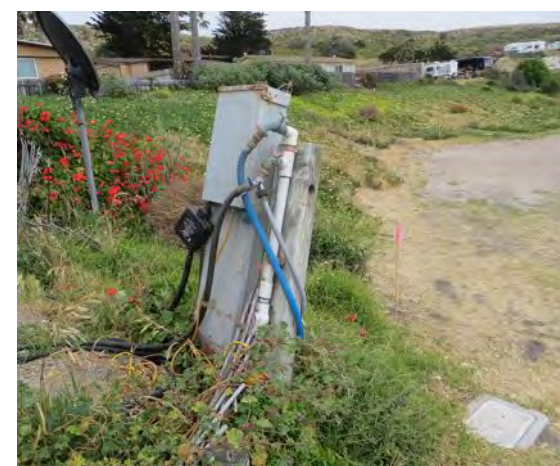
(E) hosebib & electrical pedestal by Host RV to be relocated and replaced
