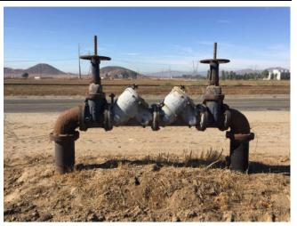
Photo 8: View of the backflow prevention plumbing located at the southern property boundary.
