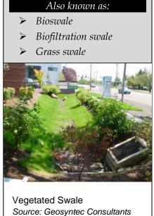
channel for dry weather flows may be required to minimize ponding and convey treated and/or dry weather flows to an acceptable discharge point. An effective vegetated swale achieves uniform sheet flow through a densely vegetated area for a period of several minutes. The vegetation in the swale can vary depending on its location within the project area and is generally the choice of the designer, subject to the design criteria outlined in this section.
