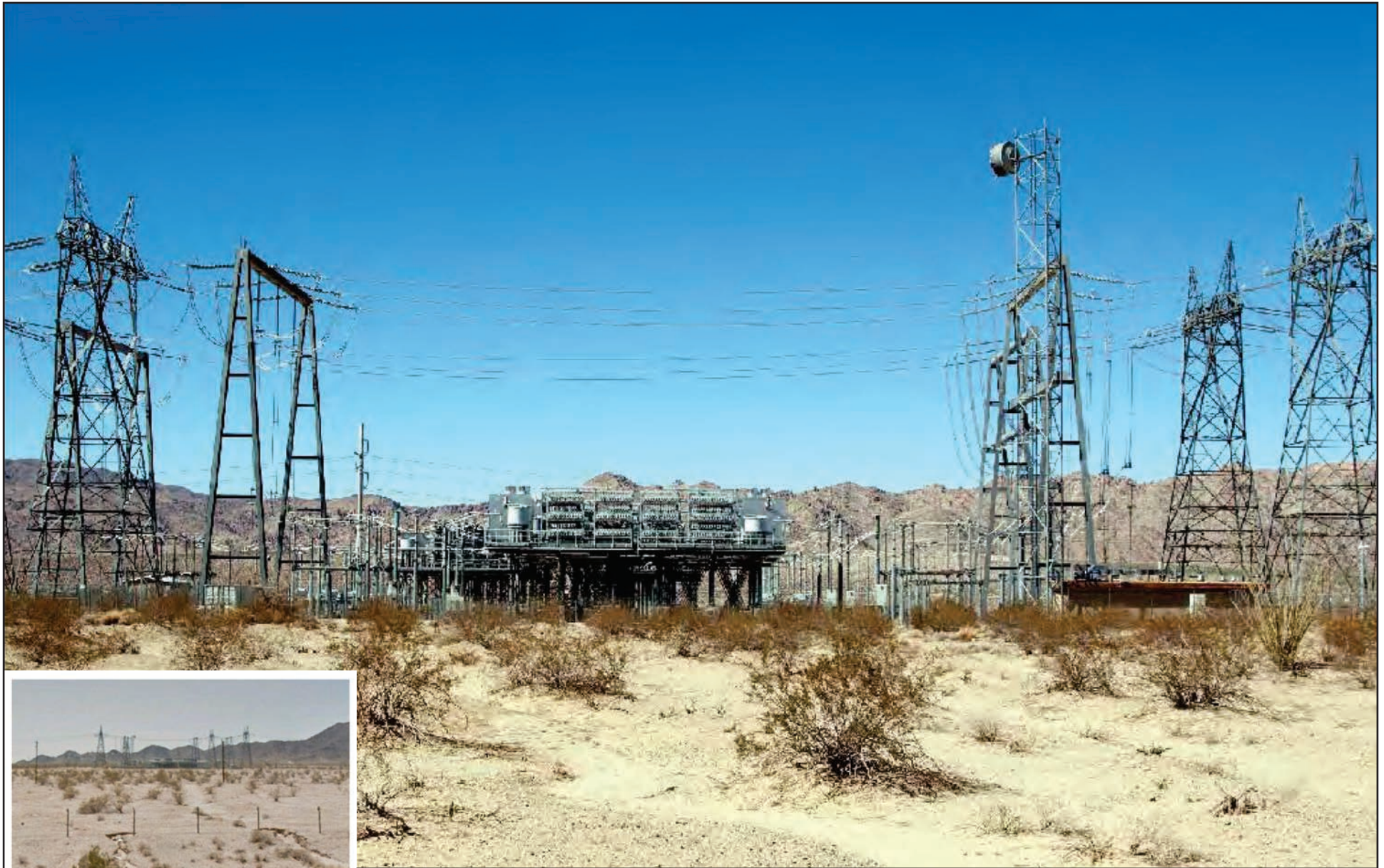
Figure 5.1-1 Devers-Red Bluff 500kV Mid-Line Capacitor
