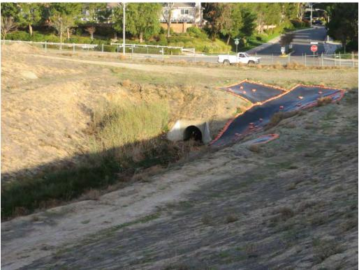
**Photograph 8:** Looking at the culvert that delivers urban and stormwater runoff from the neighborhoods to the north onto the project site.
