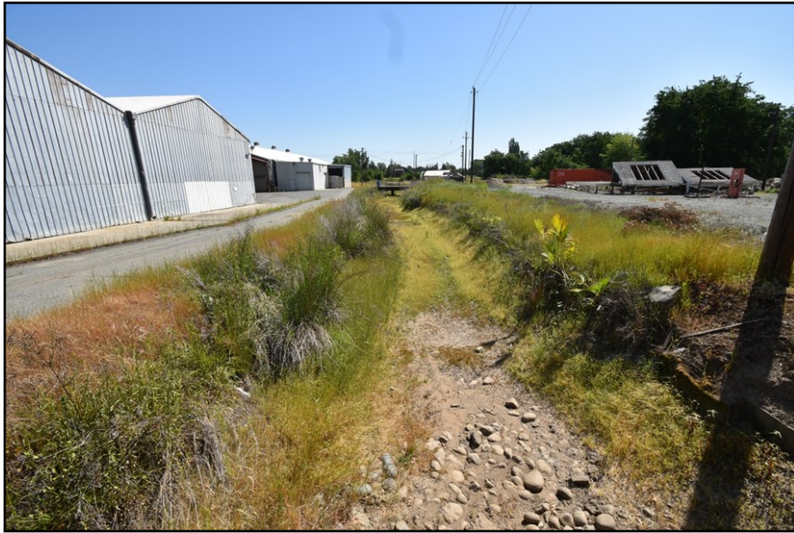
Photo 5: View looking east showing tributary ditch feature to Morrison Canal.
