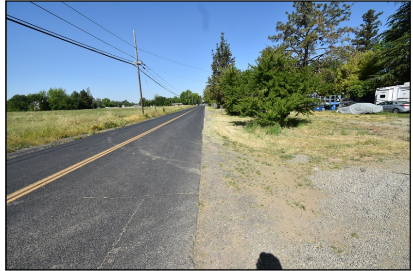
Photo 2: Looking west along the north side of Little Avenue into the work area.
