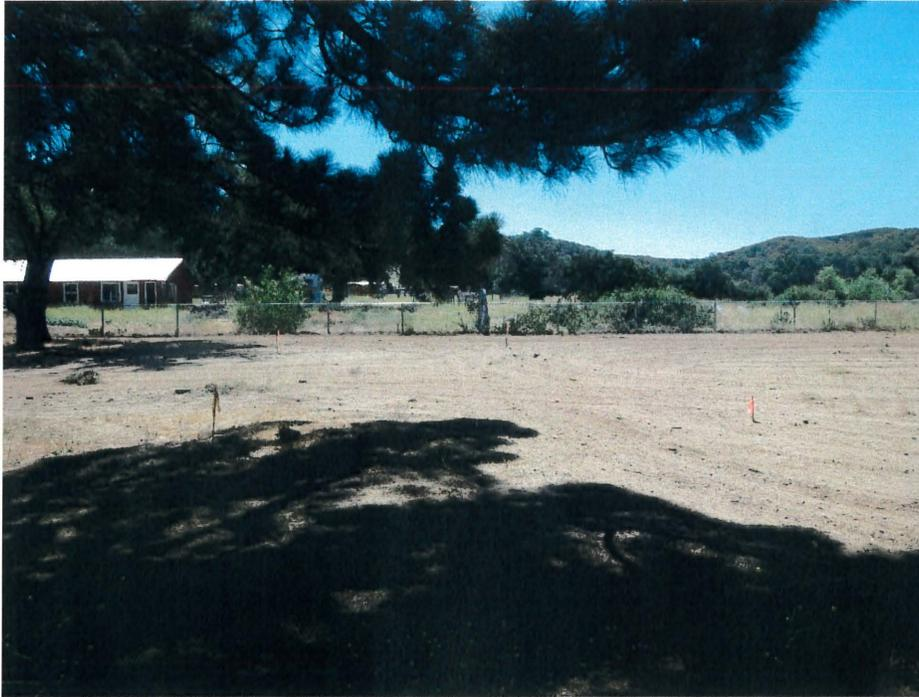
Photo #1: Looking east across location where building will be placed. Flags indicate rough location of building corners.
