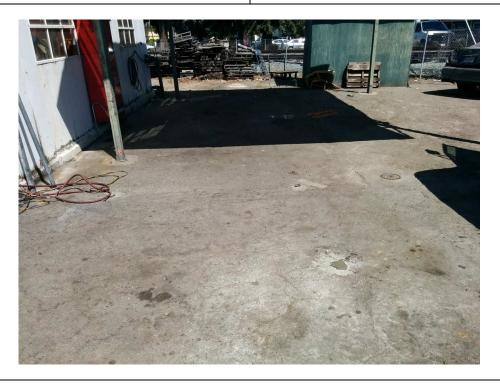
Subject: Borings backfilled, surface repaired (typical).
