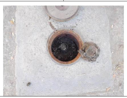
Subject: Subject Property, Fill Box observed on the south side of 1420 South Bascom (the Smog Testing Shop), It appears to be a fill spout for an underground storage tank (UST), filled with sand
