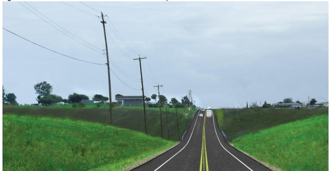
**Figure 6: KV #1** – Vertical curve correction with side slope construction.
