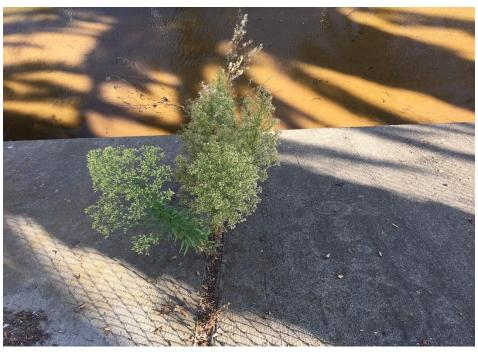
Photograph 17. Vegetation growing out of the crack between concrete slabs lining Colma Creek channel.
