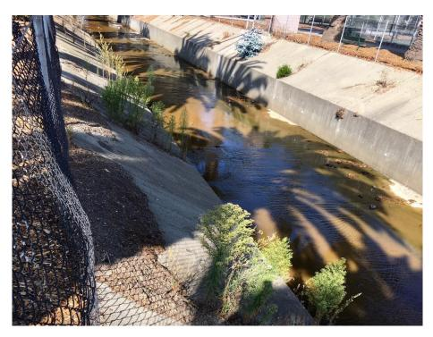
Photograph 18. Vegetation growing out of the crack between concrete slabs lining Colma Creek channel.
