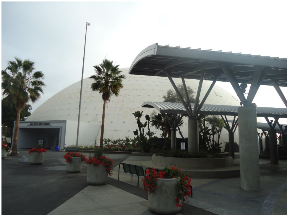
Photo 18 - Adjoining property to northeast (cruise line passenger terminal)
