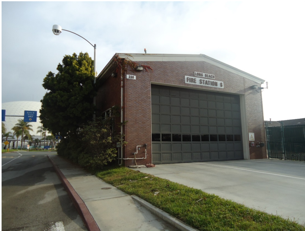
Photo 13 - Adjoining property to southeast of parking garage (fire department)
