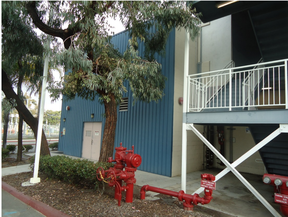
Photo 21 - EnWave Energy Power Plant adjoining northeastern side of parking garage
