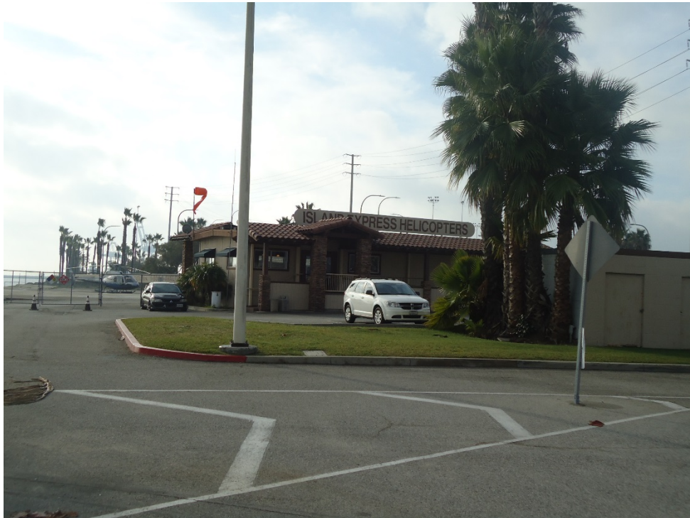
Photo 14 - Adjoining property to southeast of parking garage (Island Express Helicopters)
