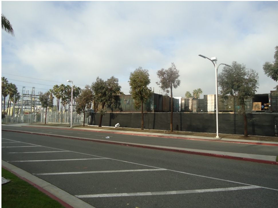
Photo 16 - Adjoining property to northwest of parking garage (parking lot with construction equipment)
