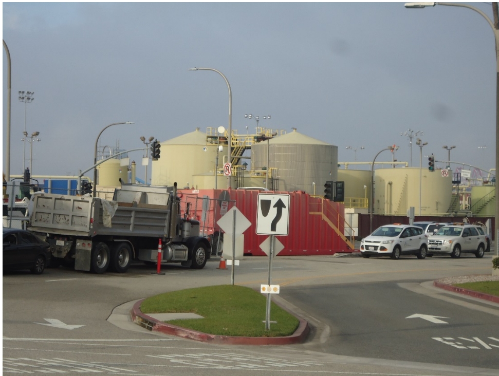
Photo 15 - Adjoining property to southwest of parking garage (bulk oil facility)
