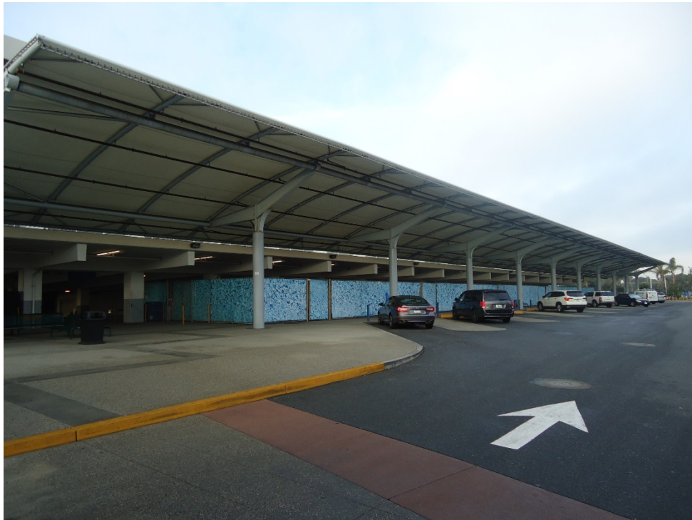
Photo 4 - View of Site parking garage - northeast side, facing west
