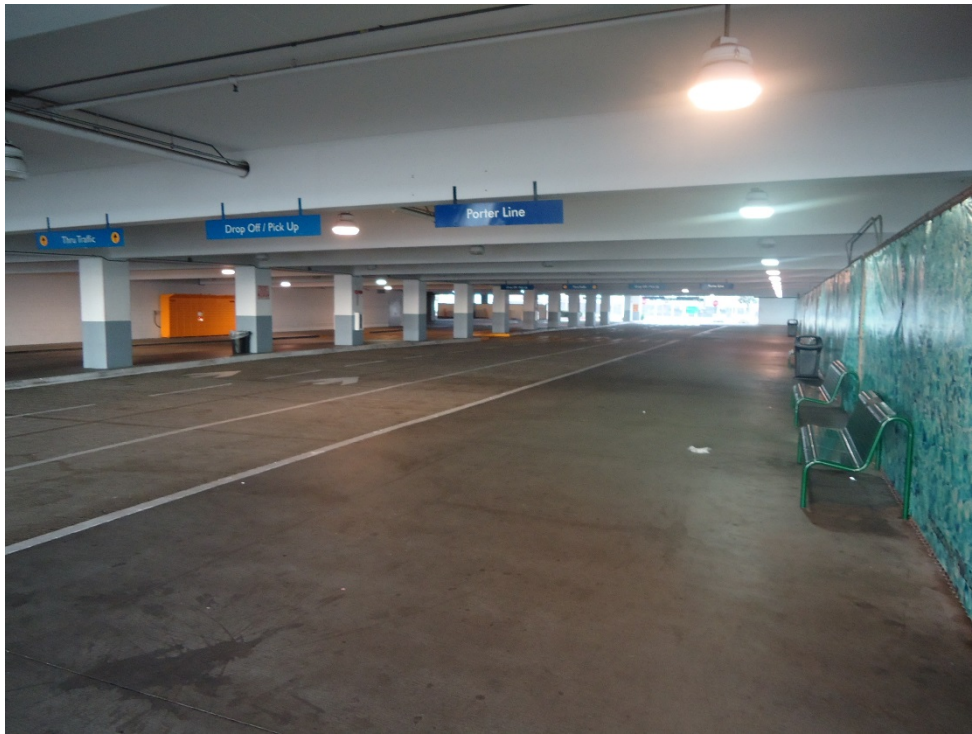
Photo 19 - Parking garage area
