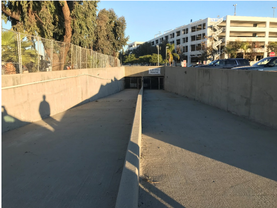
Photo 7 - South tunnel entrance
