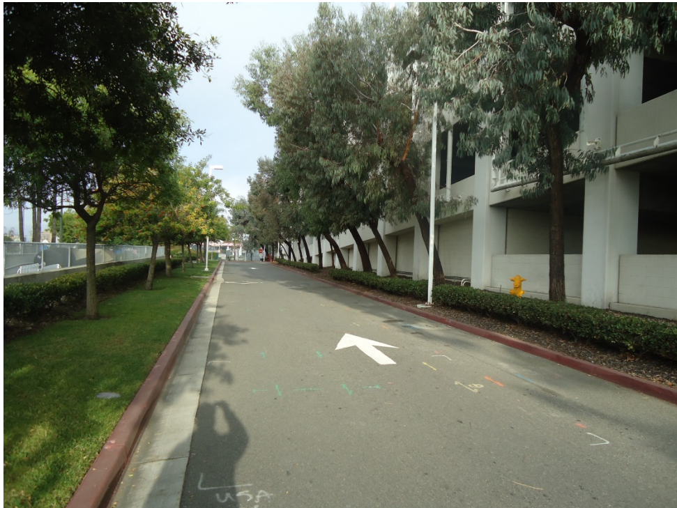
Photo 2 - View of Site parking garage - southwest side, facing northwest
