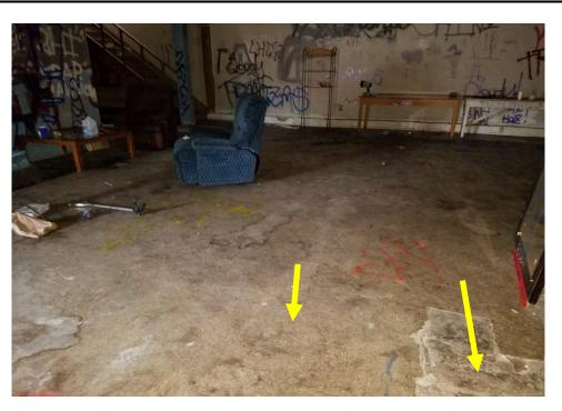
Photograph 5: Building 1: view of asbestos-containing 1'x1' vinyl floor tile and mastic.
