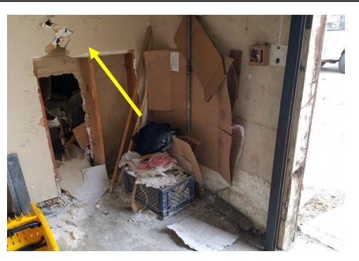
Photograph 11: Building 2: view of asbestos-containing joint compound associated with drywall.
