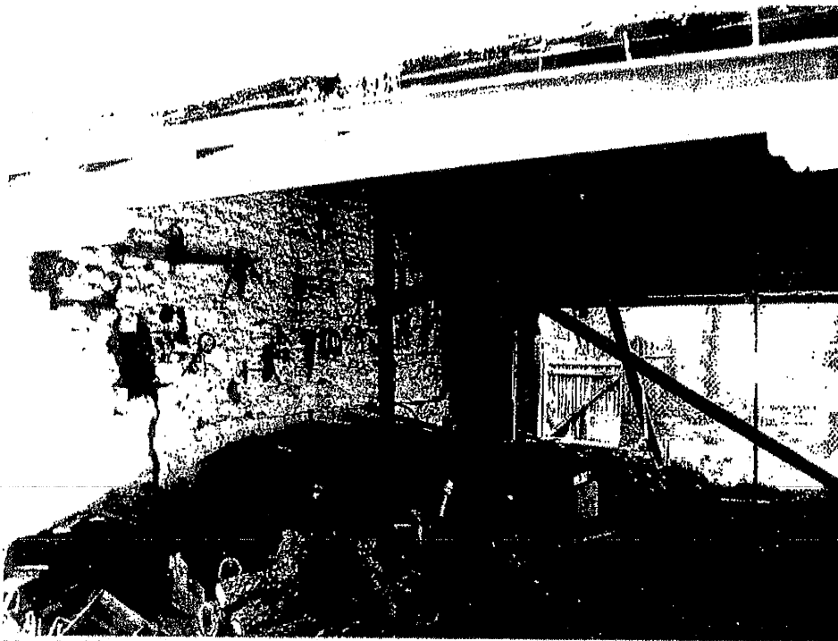
North Elevation – Cocina: Repair Corners & Replace Lower 48 inches of Adobe Wall Along Entire Length
