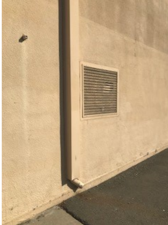
Figure 77. Exterior vent and rain gutter
