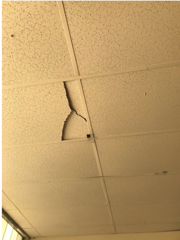
Figure 62. Minor ceiling damage
