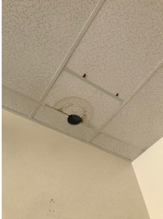
Figure 51. Former ventilation conduit
