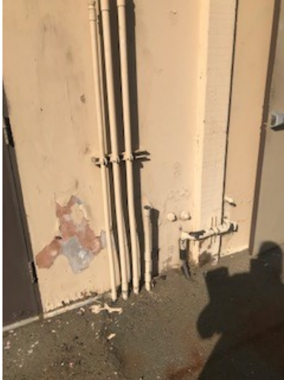
Figure 49. Paint chipping on building exterior
