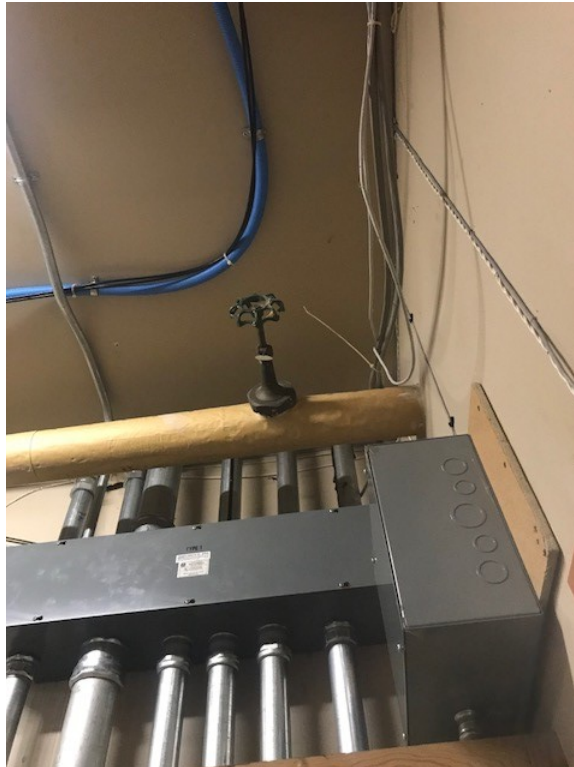
Figure 38. Electrical conduits in storage closet
