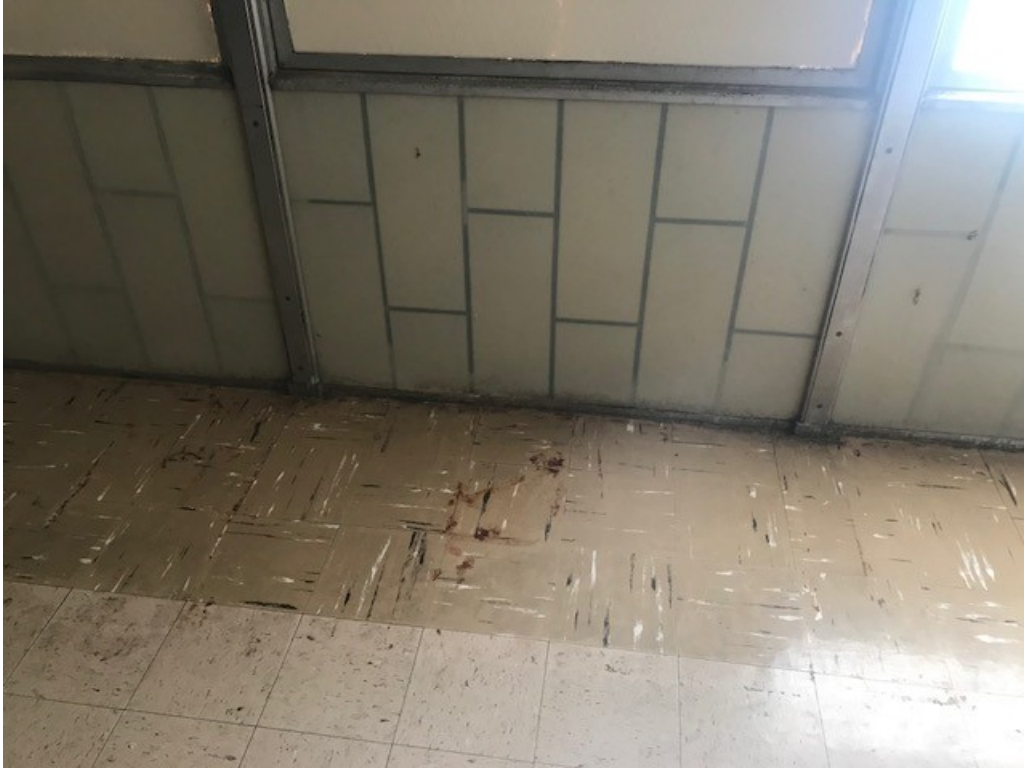
Figure 31. Change of flooring near window wall contact
