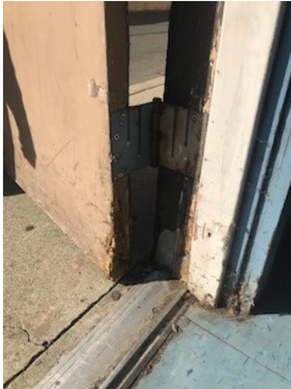
Figure 28. Degrading door from multi-purpose room to exterior
