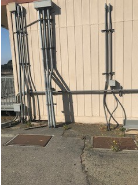
Figure 47. Electrical conduits to portable
