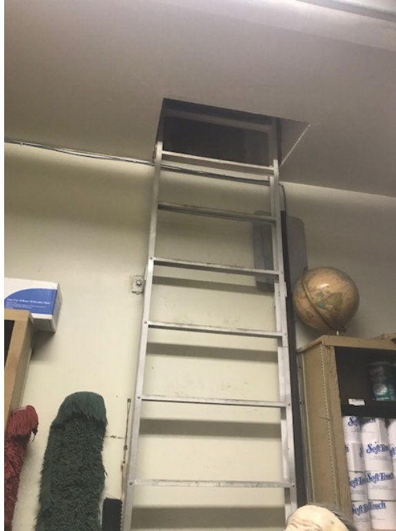
Figure 9. Roof access via stairs in custodians room
