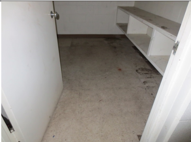
Empty office area with 9" x 9" vinyl floor tile (suspect ACM). floor tile (suspect ACM).
