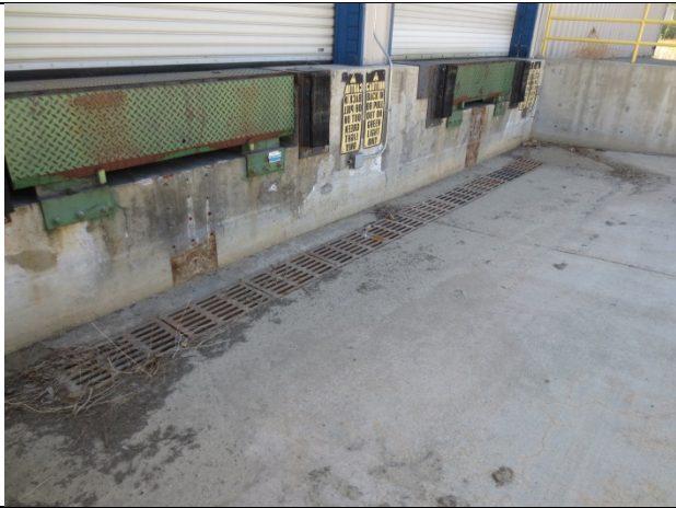
Ribbon drain at base of loading ramp.
