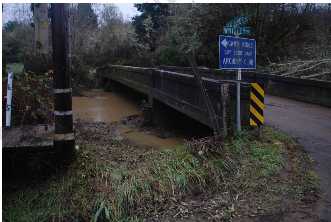
Figure 28. The mainstem Elk River in the downstream portion of the project area during December 2014. Note flooding caused by excessive fine sediment aggradation.
