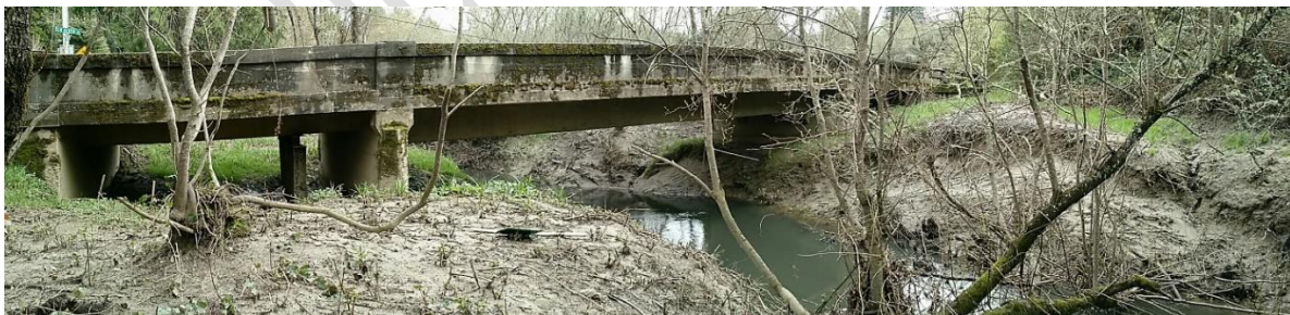
Figure 13. Fine sediment deposits at the upstream side of the Elk River Road concrete bridge (photo point 10 on Figure 11).
