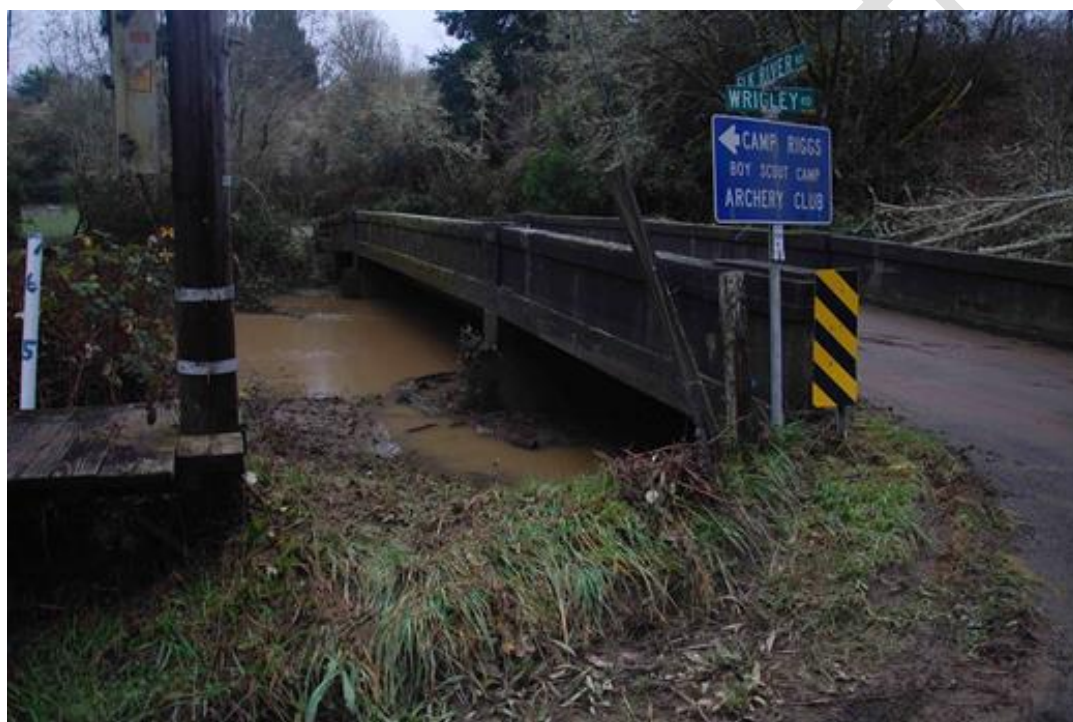
Figure 14. Mainstem Elk River at the location of the Concrete Bridge at the intersection of Elk River Road and Wrigley Road following flooding in December 2014 caused by excessive fine sediment aggradation. Note the proximity of the channel to road infrastructure.
