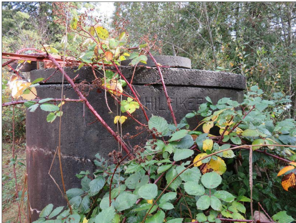
Photo 8. Closer view of the concrete springbox, stamped "HILFIKER", 11/10/2017.
