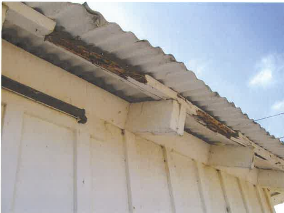
Figure 59. Deterioration of sleepers at roof framing system.
