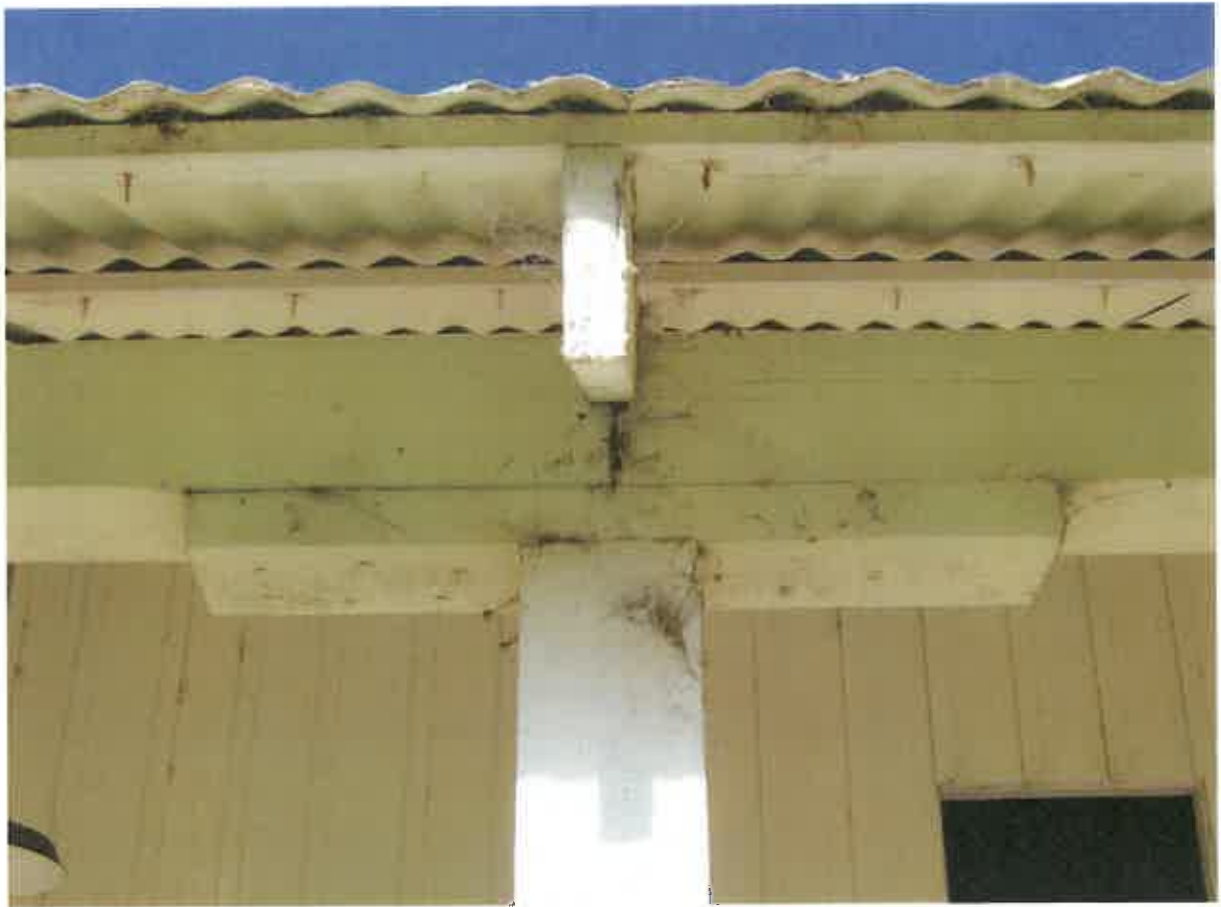
Figure 34. Structural framing system of the east aisle.
