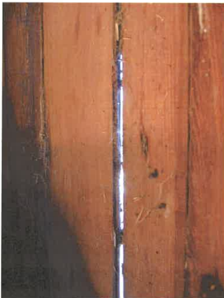
Figure 51. Typical gap between exterior siding.
