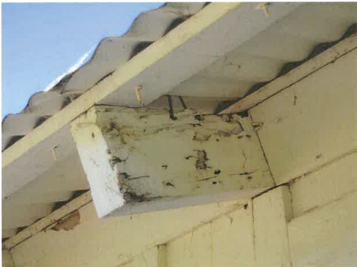
Figure 58. Typical deterioration of roof rafter ends.
