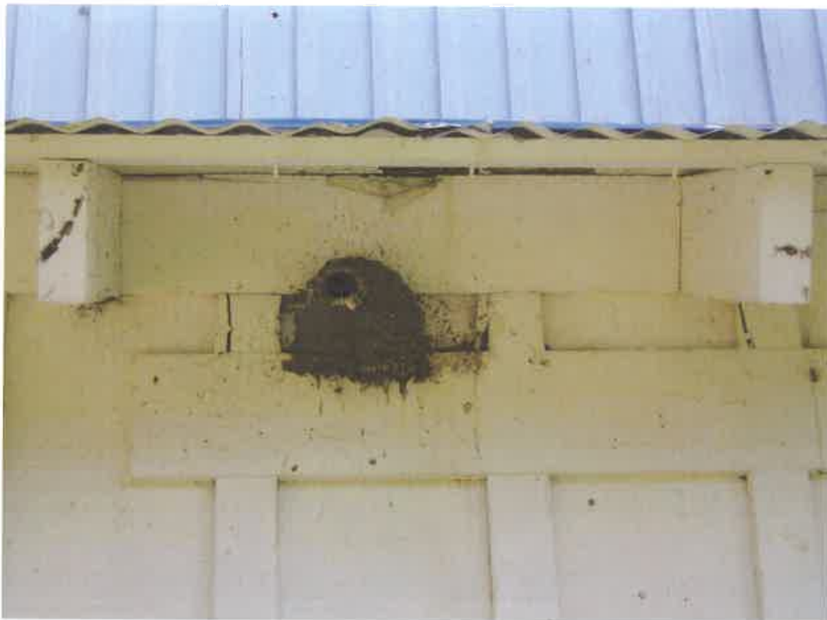
Figure 49. Bird nest found near the roof framing system at the exterior south elevation .
