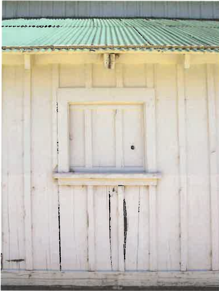
Figure 23. Typical sliding window at the west elevation.
