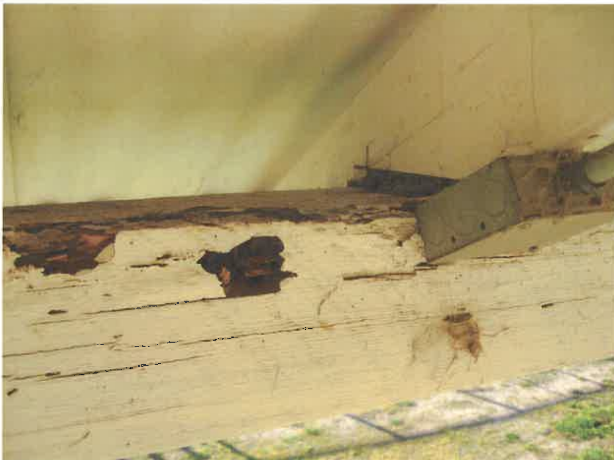
Figure 61. Deterioration of roof framing system at the east aisle caused by pests.
