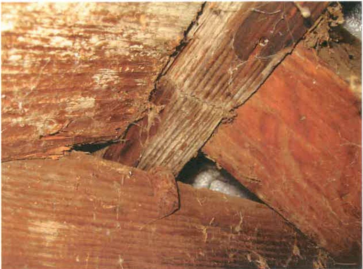
Figure 56. Deterioration at the roof framing system.
