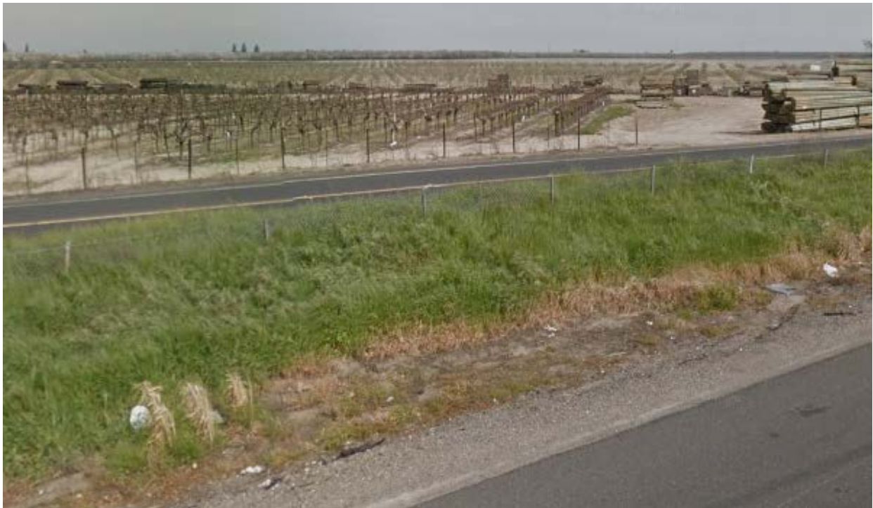
Photo 6: Frontage road parallel to SR 99 northbound.
