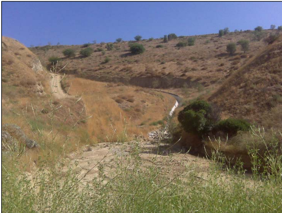
Typical view of canyon floor looking north toward the edge of the Landfill. Erosion is slowed by modern riprap and concrete channels.
