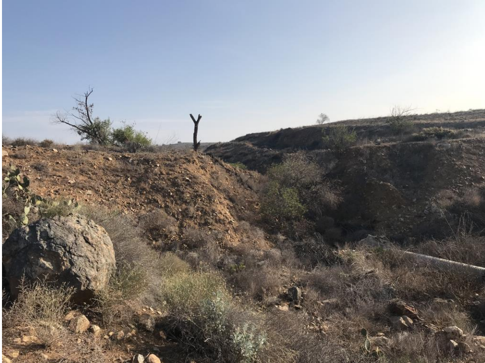
Large earthen dam (left) constructed to hold water and culvert in original drainage.
