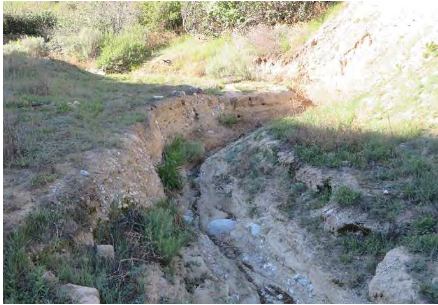
Photo 9: Feature 5 (facing downstream/south). Small and incised tributary of Feature 5 showing typical characteristics of the upper watershed.
