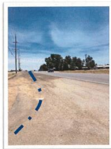
Figure 2 Existing Condition water flows from road north and west along Avenue N towards this first outlet along Ave. N. Blue line denotes flow path
