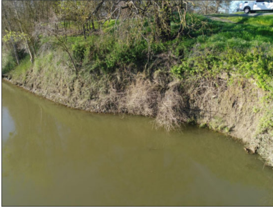
View looking southwest at vertical erosion in levee.
