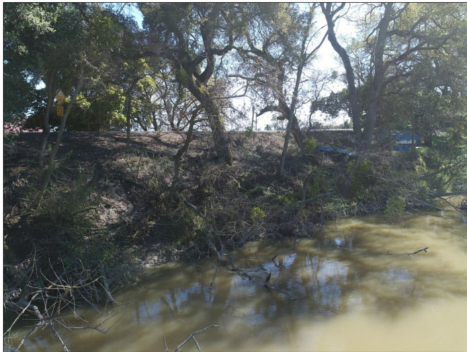
Aerial view looking southwest at erosion along waterside levee slope.
