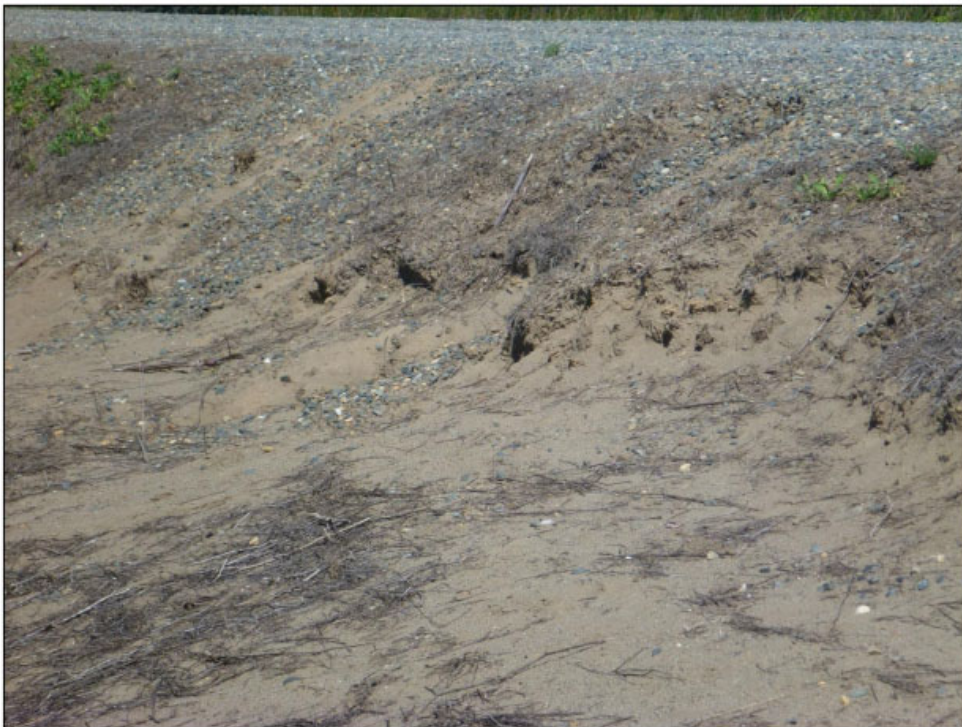
View of erosion and animal burrows along levee slope.
