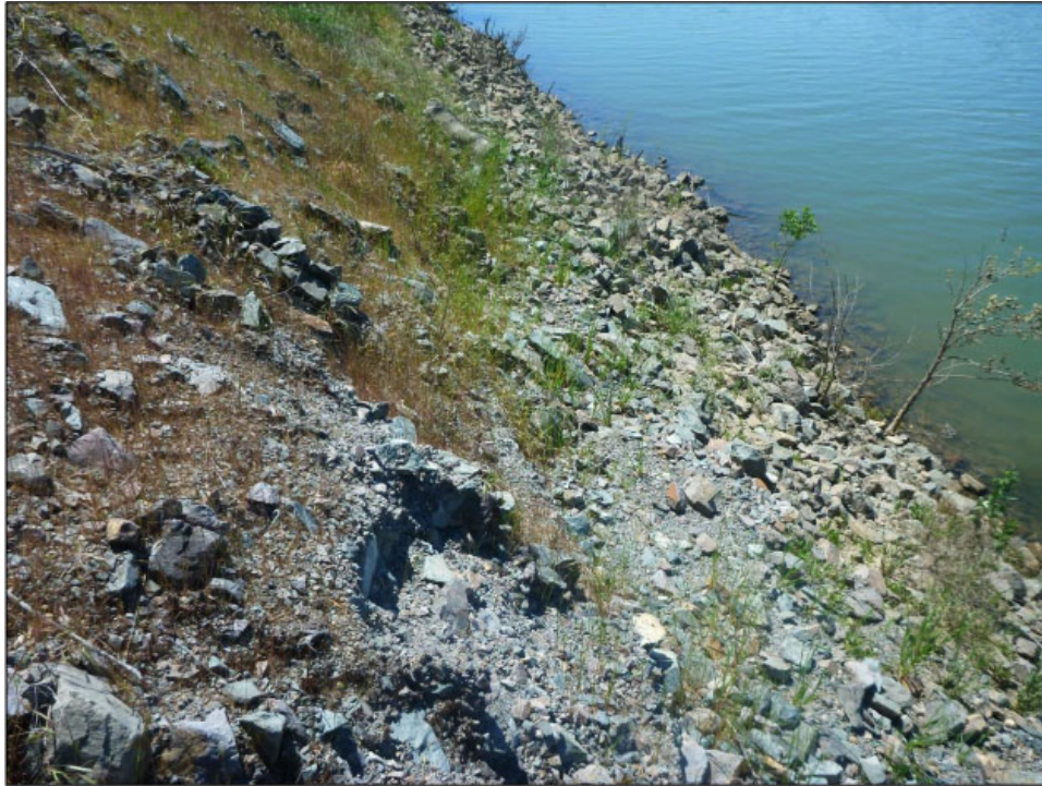
View of erosion along waterside levee which has fallen to the levee toe.
