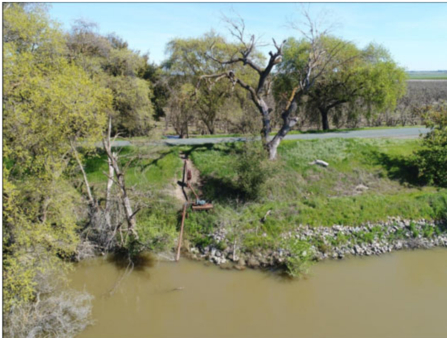
Aerial view looking at water intake pipe, rock slope protection, and dead trees in erosion damage site.
