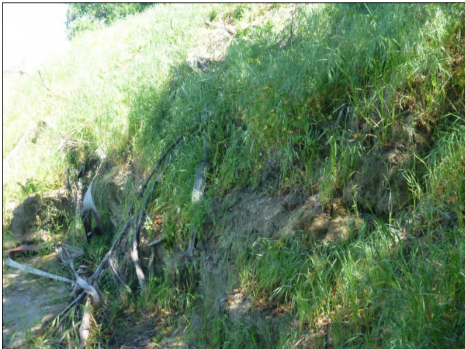
View of waterside levee slope where erosion damage exists.
