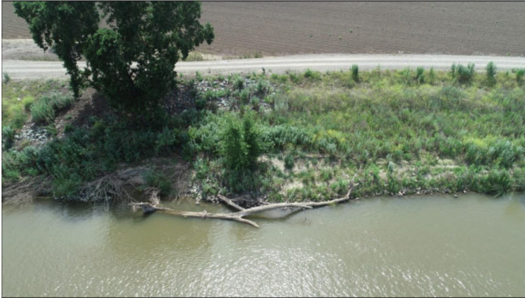
Aerial view of erosion along waterside levee slope. Emergency rock repairs visible beneath existing tree.
