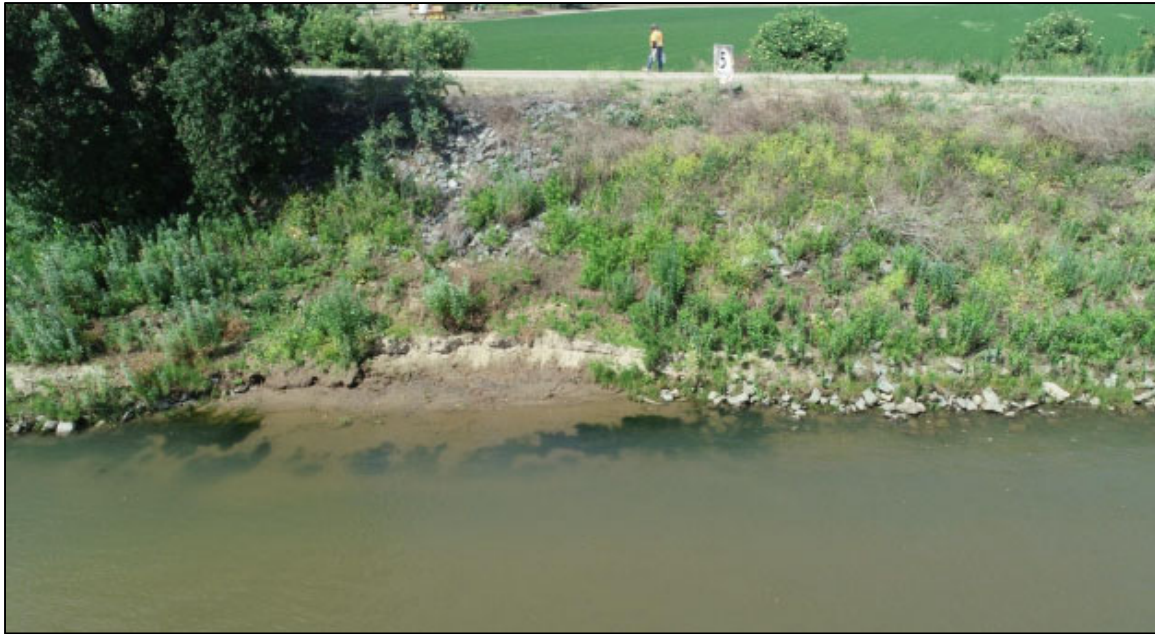
Aerial view of erosion with rock placement along waterside levee toe.
