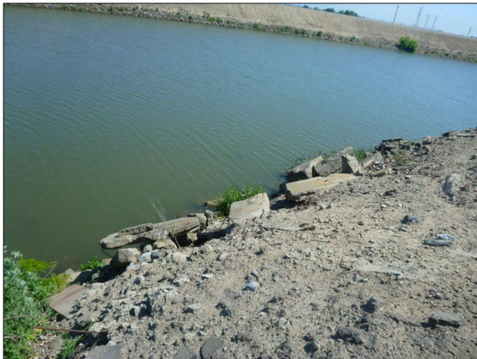
View of bank loss and construction debris
