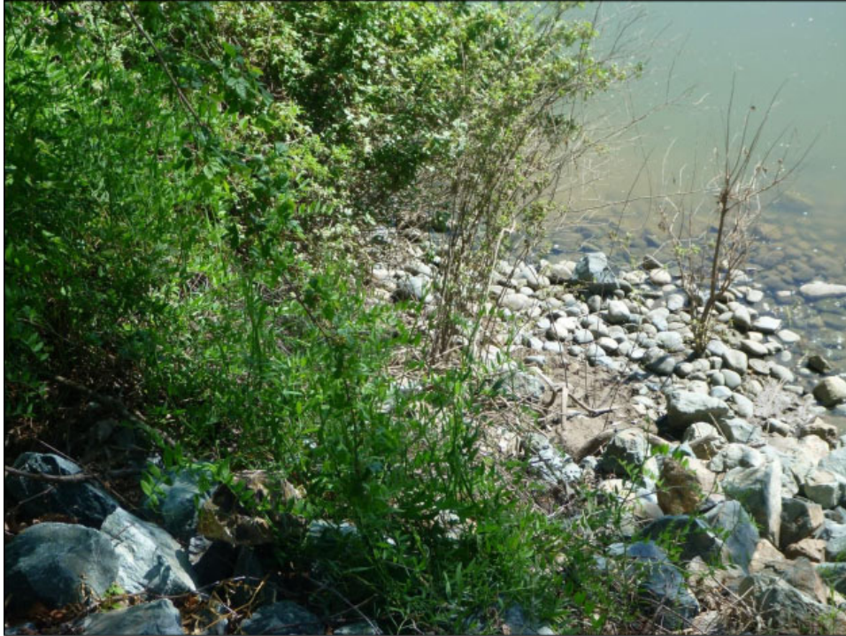
View of erosion and rock placement from emergency erosion repairs visible along waterside toe.
