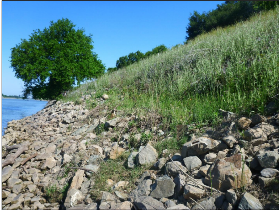
View of waterside levee erosion rock placement repair.
