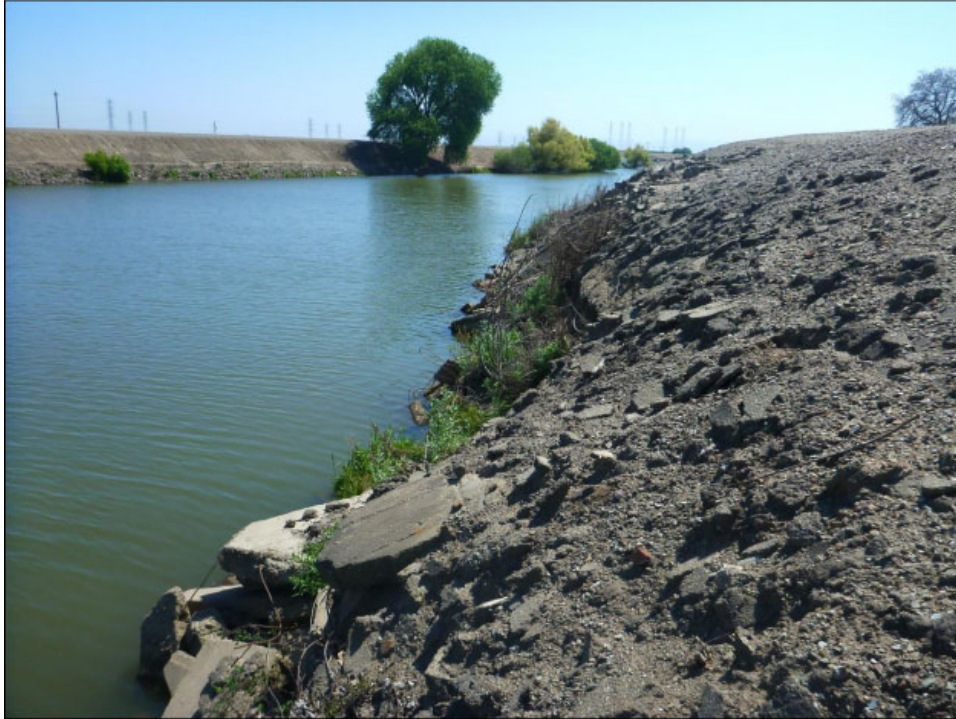
View looking south of eroded bank with construction debris along waterside levee slope.
