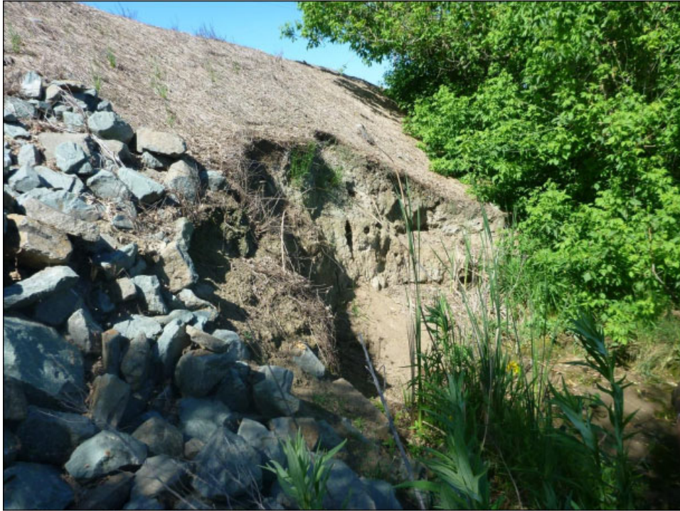
Close up view of erosion on waterside levee bank and loss of waterside toe.
