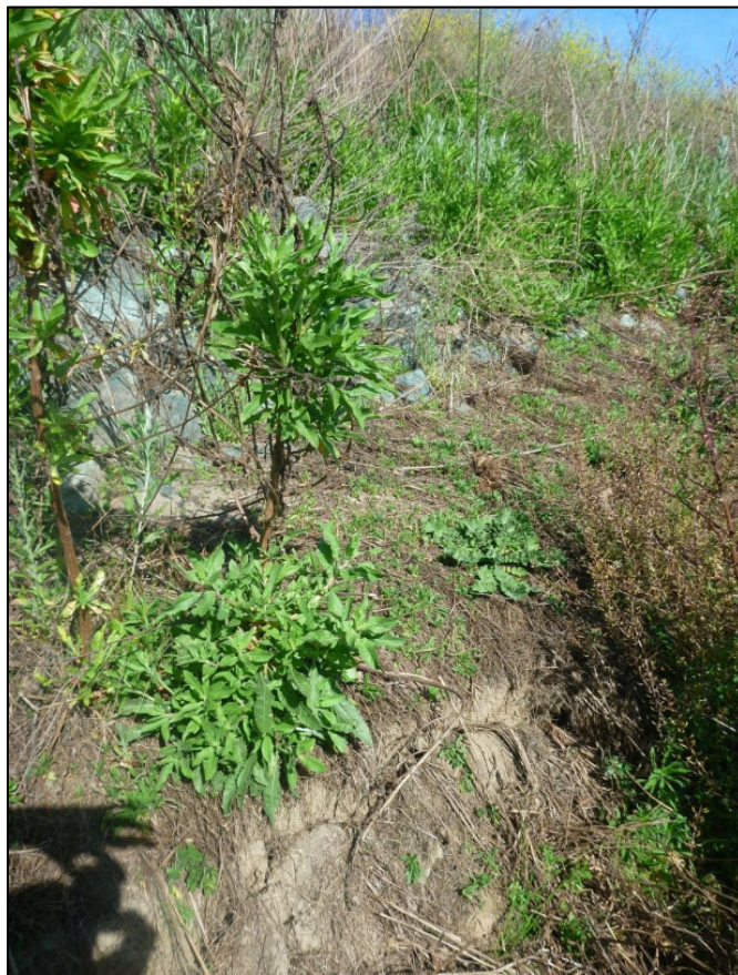
View of rip rap repair above erosion along waterside levee slope.
