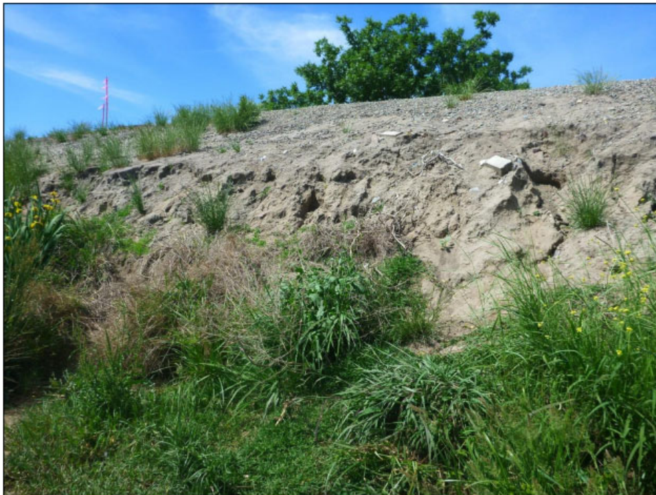
View of waterside erosion, continues throughout the entire repair site.
