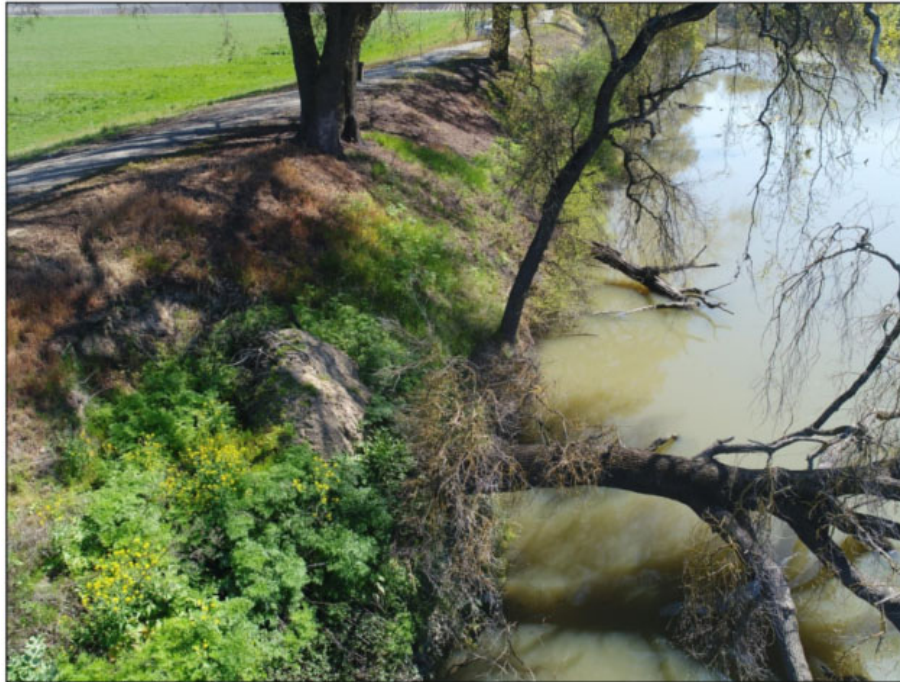
Aerial view of erosions damage site. Hole in bank left by root ball is obscured by vegetation.
