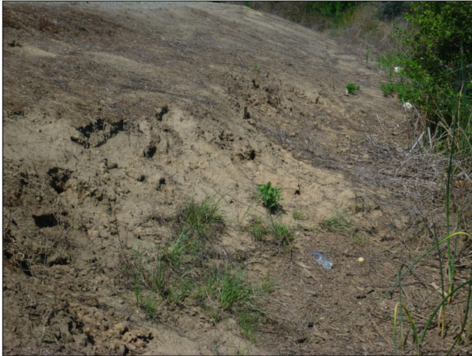
View of erosion along waterside levee slope.
