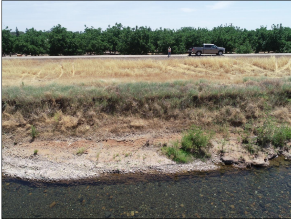
Bank erosion at damaged site.
