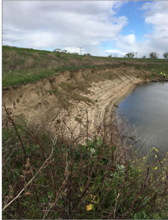
View looking from upstream at waterside levee bank erosion.
