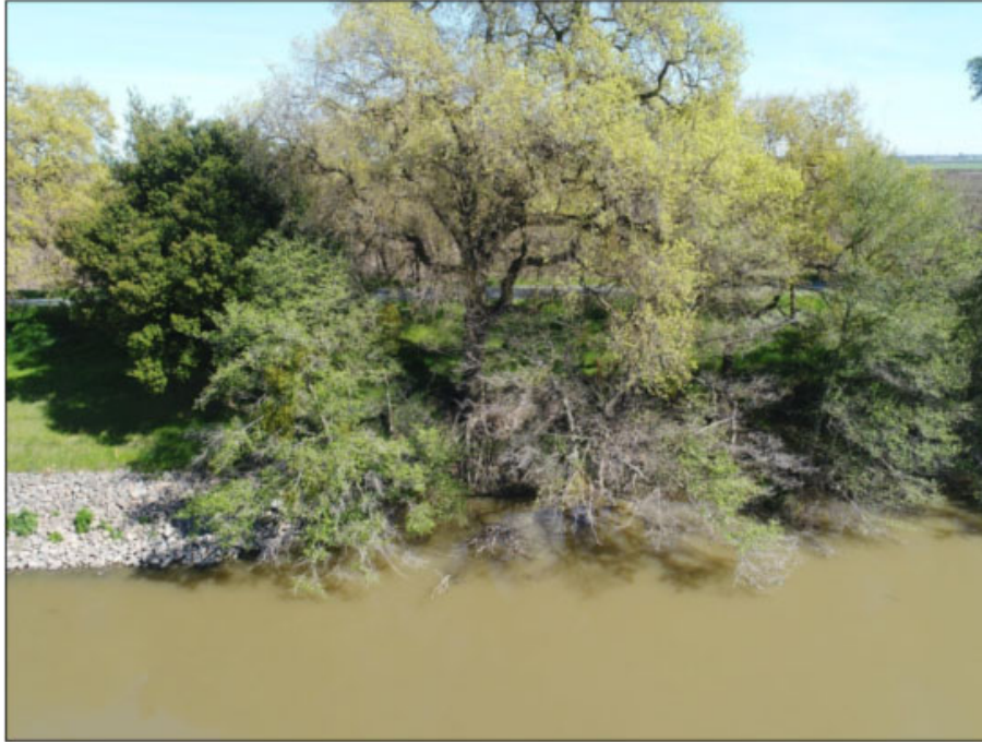
Aerial view of waterside levee slope looking at the upstream end of the erosion damage site. Erosion damage begins at the end of the rock protection, visible on the left side of the photo, placed during emergency repairs.
