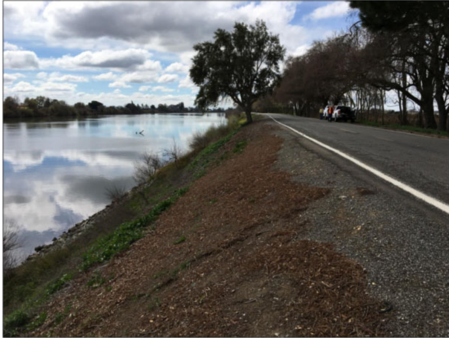
View of repair site with rock slope protection visible along water side levee toe. Cracking of highway pavement appears to be associated with the levee erosion damage.
