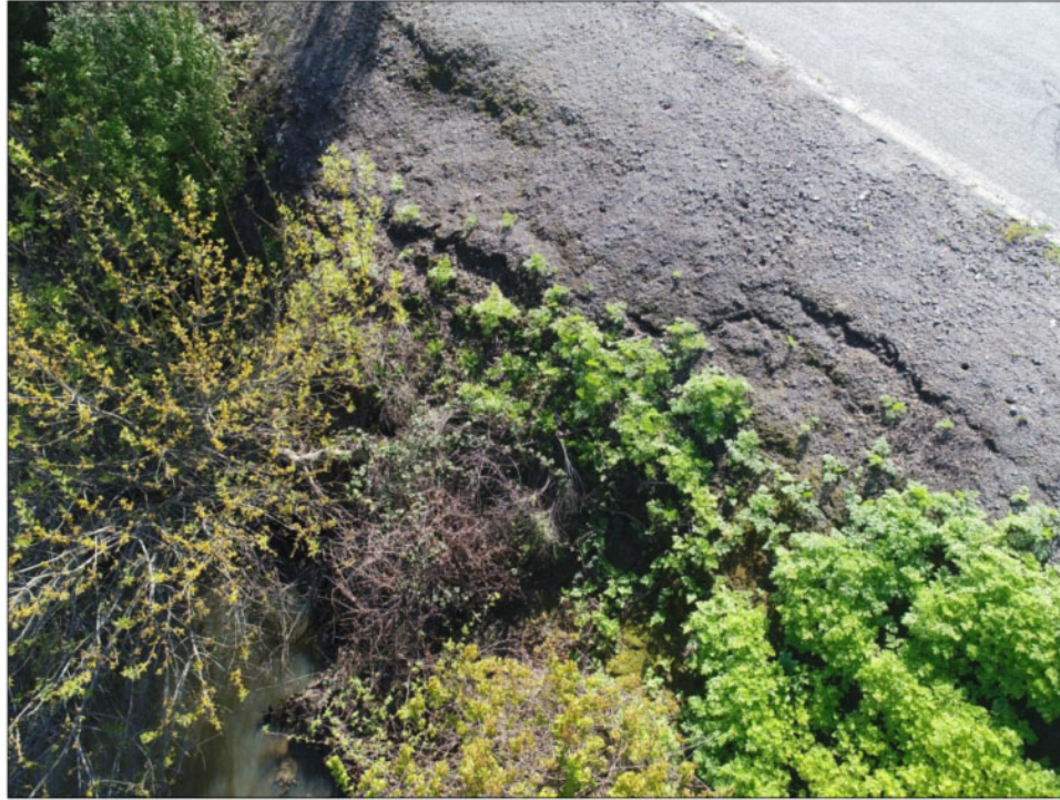
View of bank slope erosion and associated cracking of road along levee crest.
