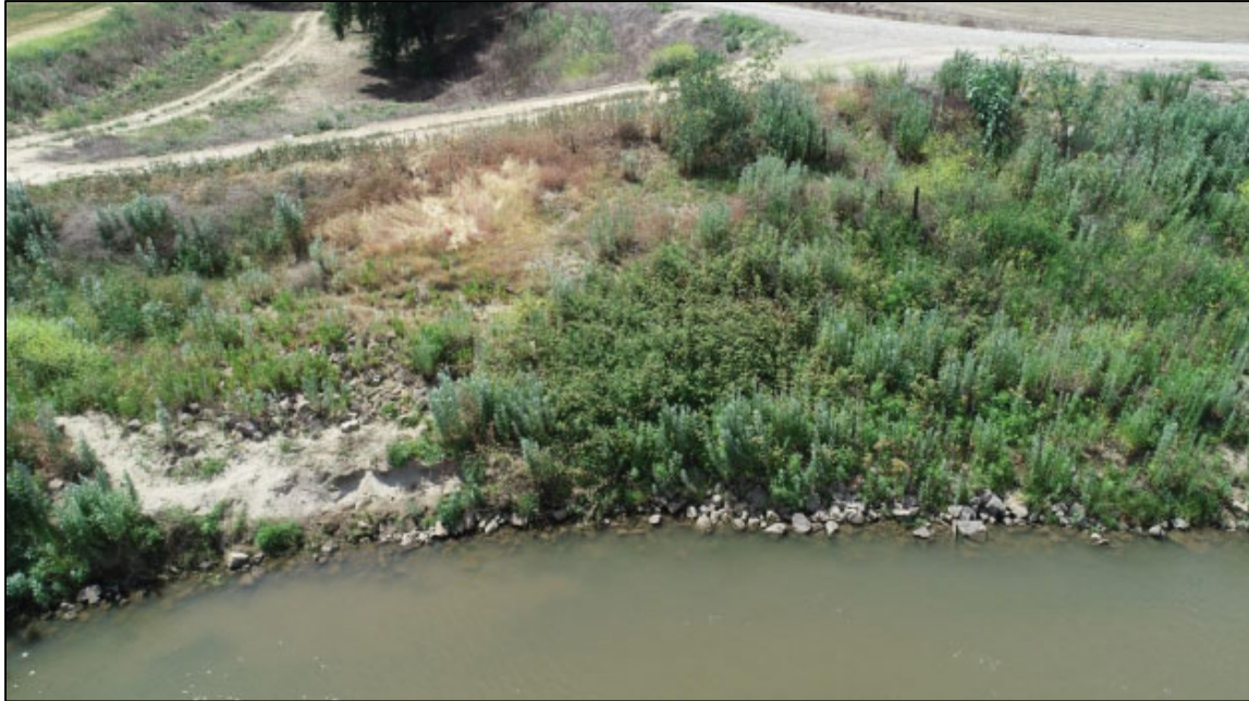
Aerial view of erosion with rock repair armoring longitudinally along repair site.
