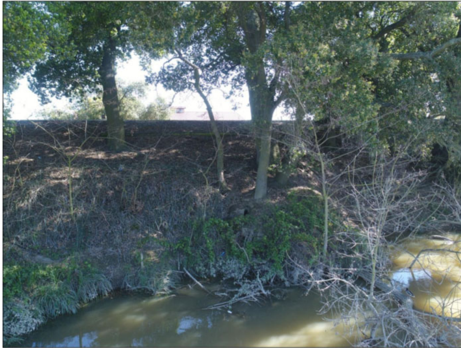
Aerial view looking south at waterside levee slope. Downed tree visible in foreground.
