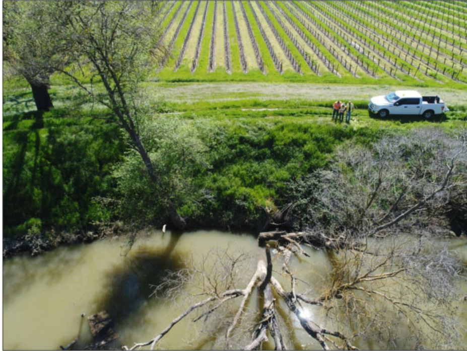
Aerial view looking at southern levee slope erosion damage. Erosion damage has felled the tree and exposed the levee to more erosion around the root ball hole.
