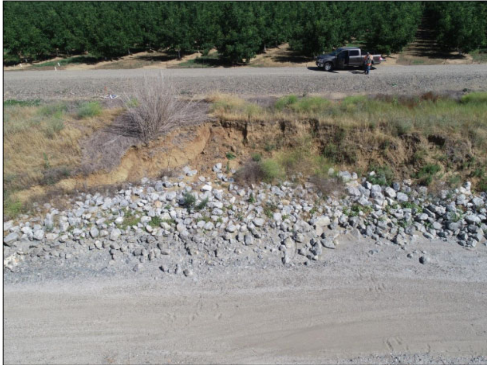
Aerial imagery of erosion and emergency rock repair at the damaged site.
