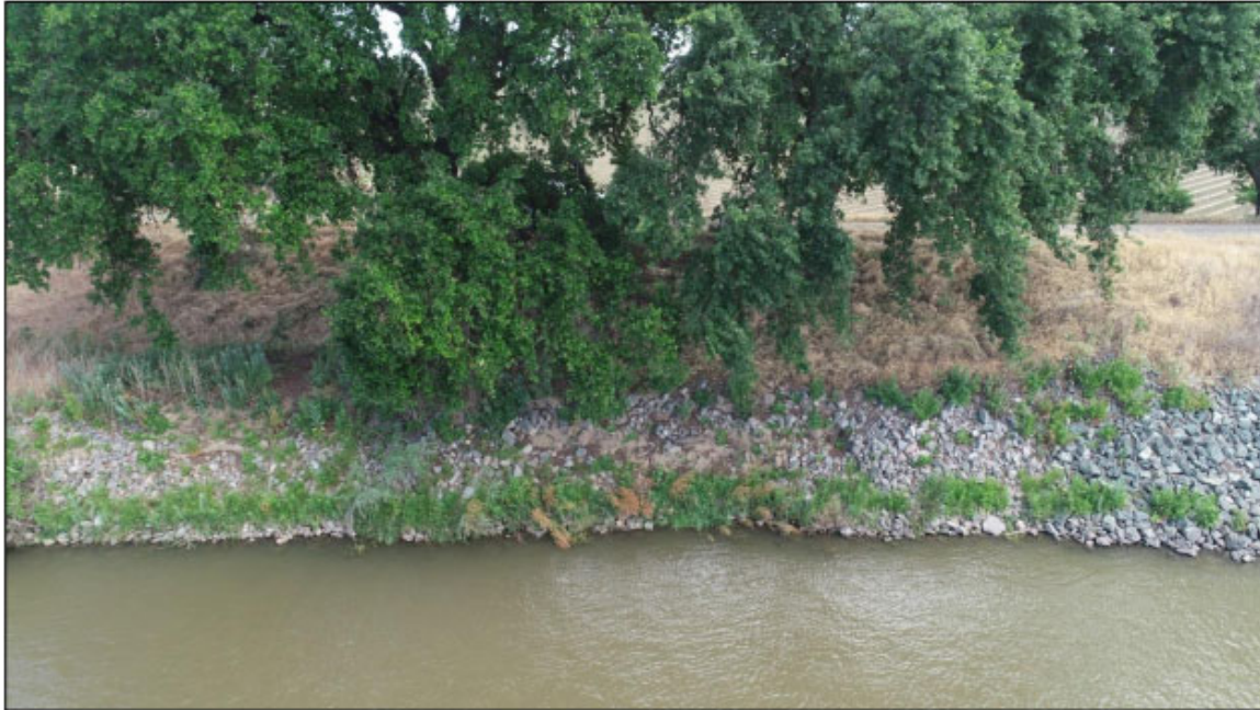
Aerial view of erosion and emergency rock placement repair under tree.
