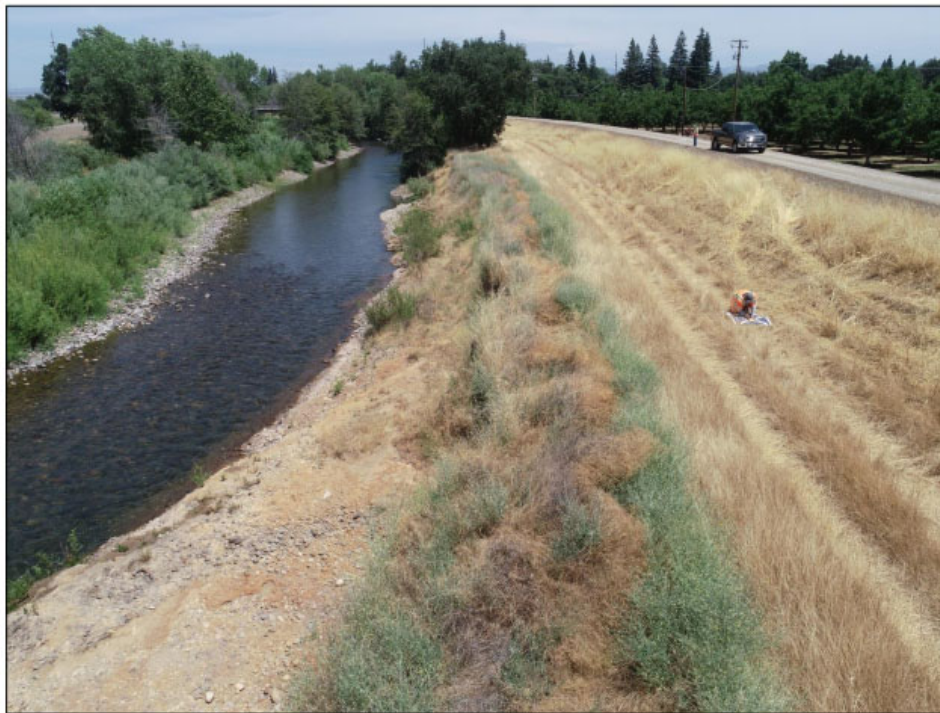
View looking upstream of erosion along southern levee slope.
