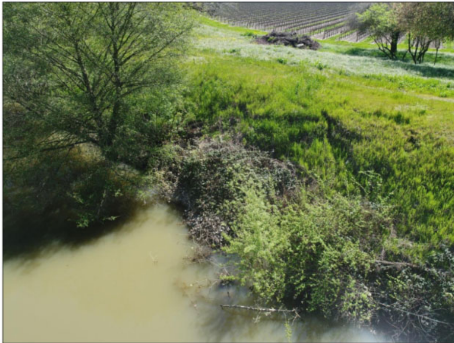
Tension cracking, visible as shadows in the waterside levee slope vegetation.
