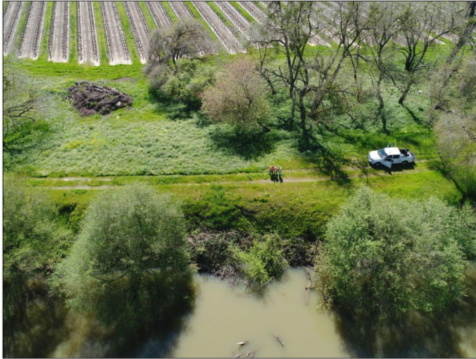
Aerial view looking at southern levee waterside slope erosion damage. Erosion scarp and tension cracking have working into the levee prism and are beginning to encroach on the levee crest.
