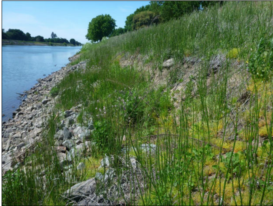
View of waterside levee toe erosion above emergency rock repair.
