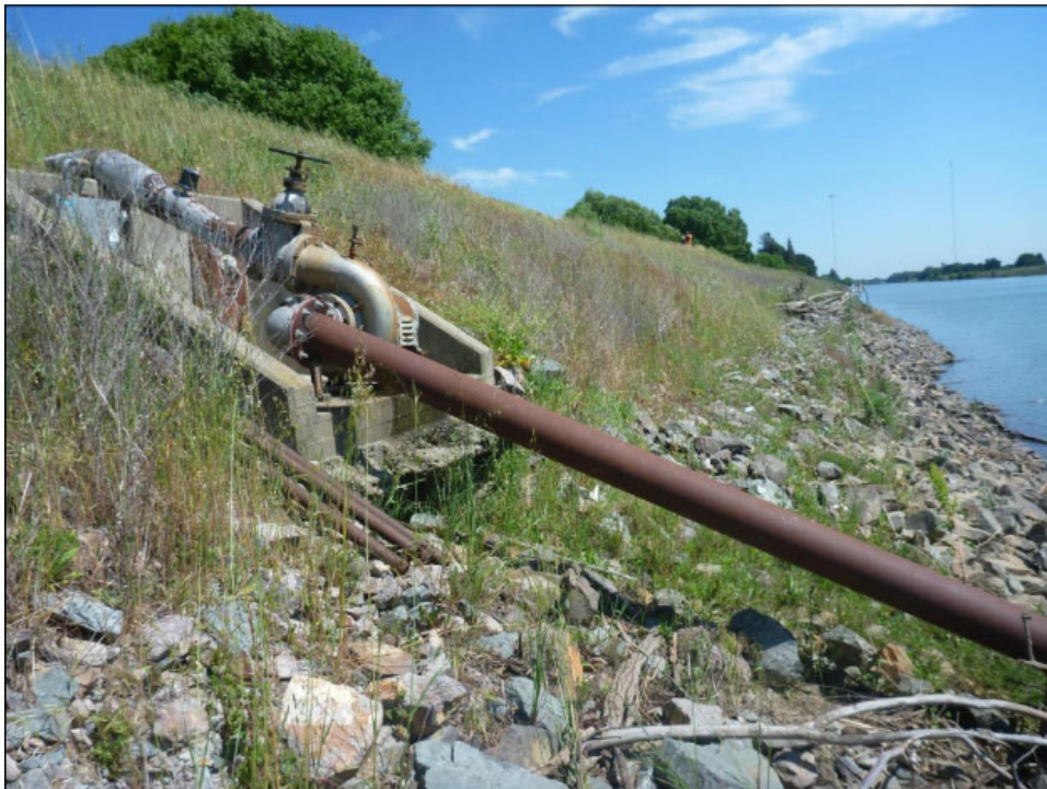
View of levee slope depression beneath pipe structure and emergency rock repair along levee waterside toe.
