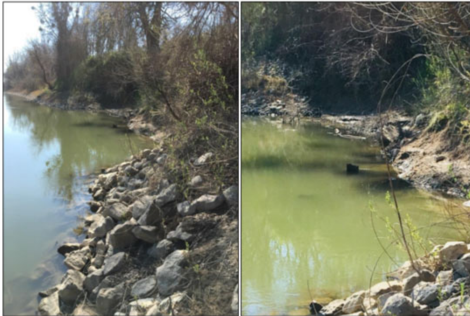
Left. Downstream view of erosion and emergency rock repair at damaged site. Right. Exposed H-pile protruding from water approximately 4-feet from erosions site shoreline. H-pile may be part of submerged water intake structure and is submerged at higher flows.
