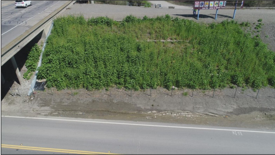
Landside erosion site after interim emergency repairs. Straw waddles for surface erosions control are visible through vegetation.
