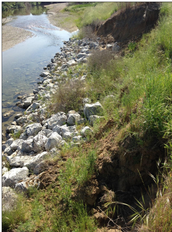
Bank erosion and emergency rock repair at the waterside toe of damaged site.
