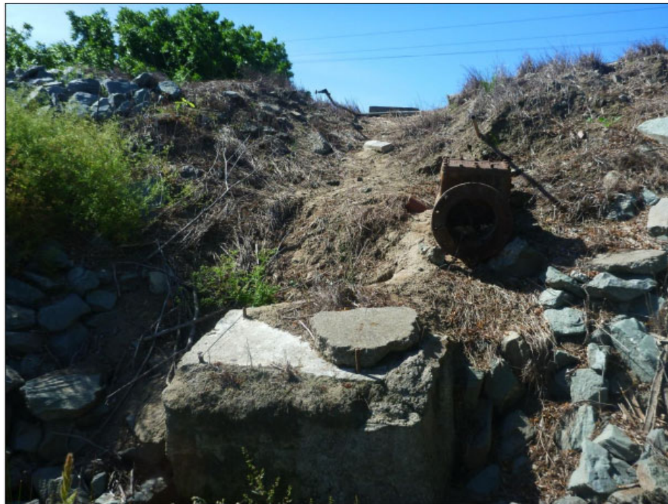
View of piping, rip rap, construction debris, and storm water erosion adjacent to repair
