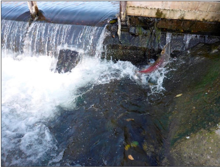
Figure 7. This fall run Chinook salmon was observed struggling to pass upstream over the concrete dam with flashboards removed. After a few attempts, the salmon was observed swimming back downstream.
