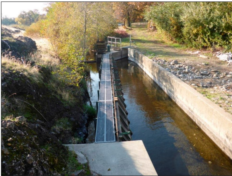
Figure 8. Existing DCID fish screen bay looking downstream from the headgates. The entrance to the juvenile bypass pipe is near the handrail at the far end of this photo.
