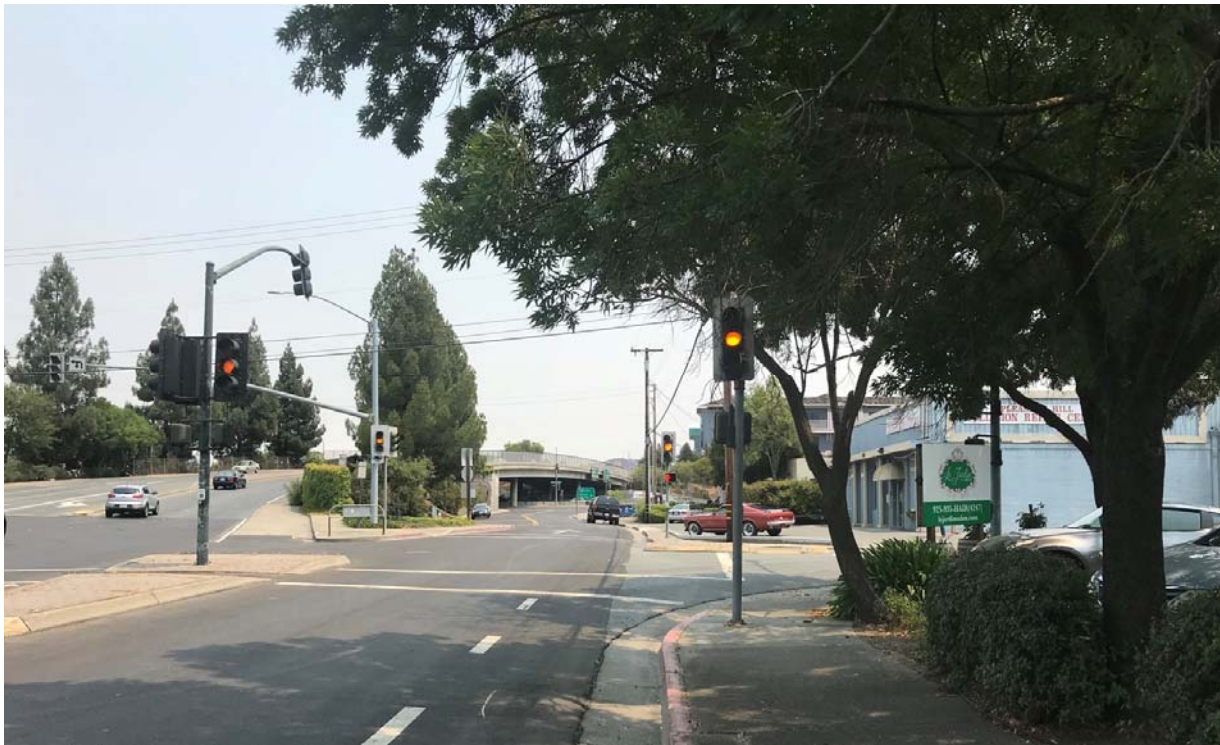
Figure 4.3b: Views of the Proposed Project from Camera 2
