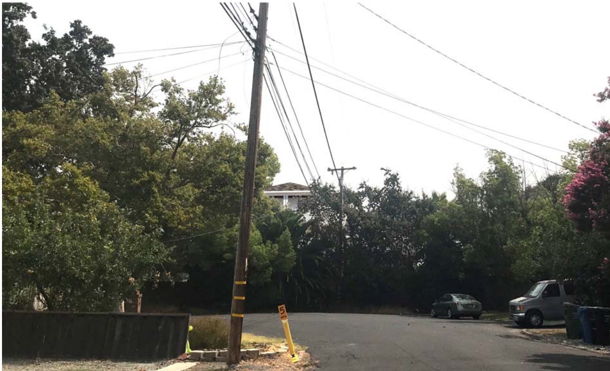
Figure 4.5b: Views of the Proposed Project from Camera 4
