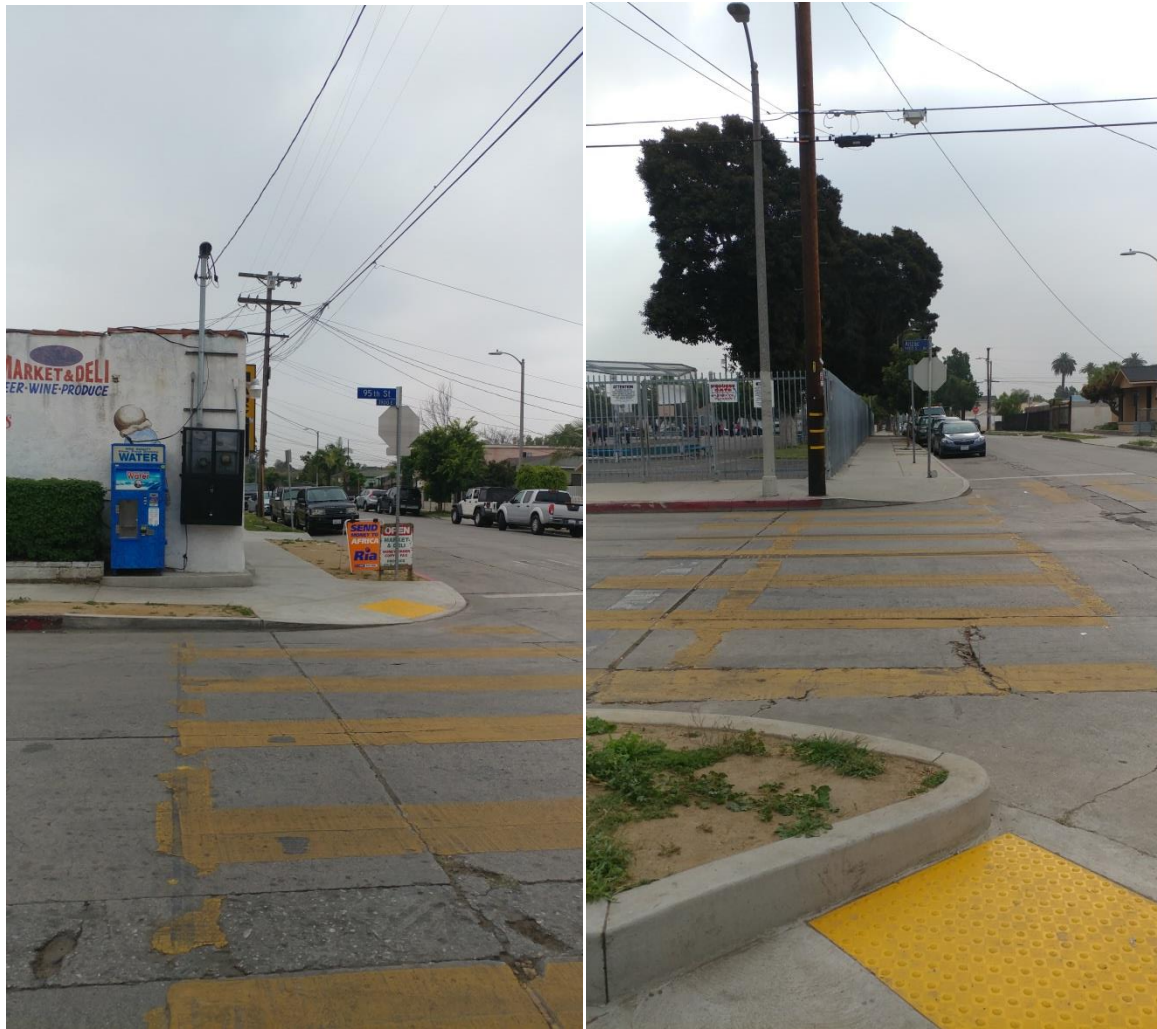
Crosswalk striping worn at the east leg (left) and crossing pavement worn and uneven at the north leg of the intersection of Anzac Ave and 95th Street
