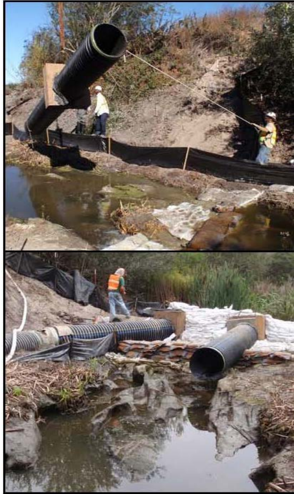
Figure 2-7. Installation of Concreted Collared Culvert.
