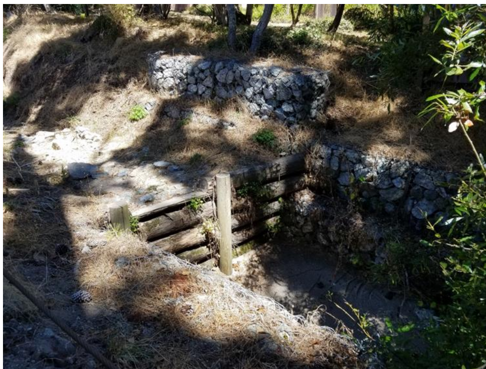
Photograph 10. Site 8, Existing log drops and gabions in upstream reach of the channel above Culvert E03-H3, facing west.
