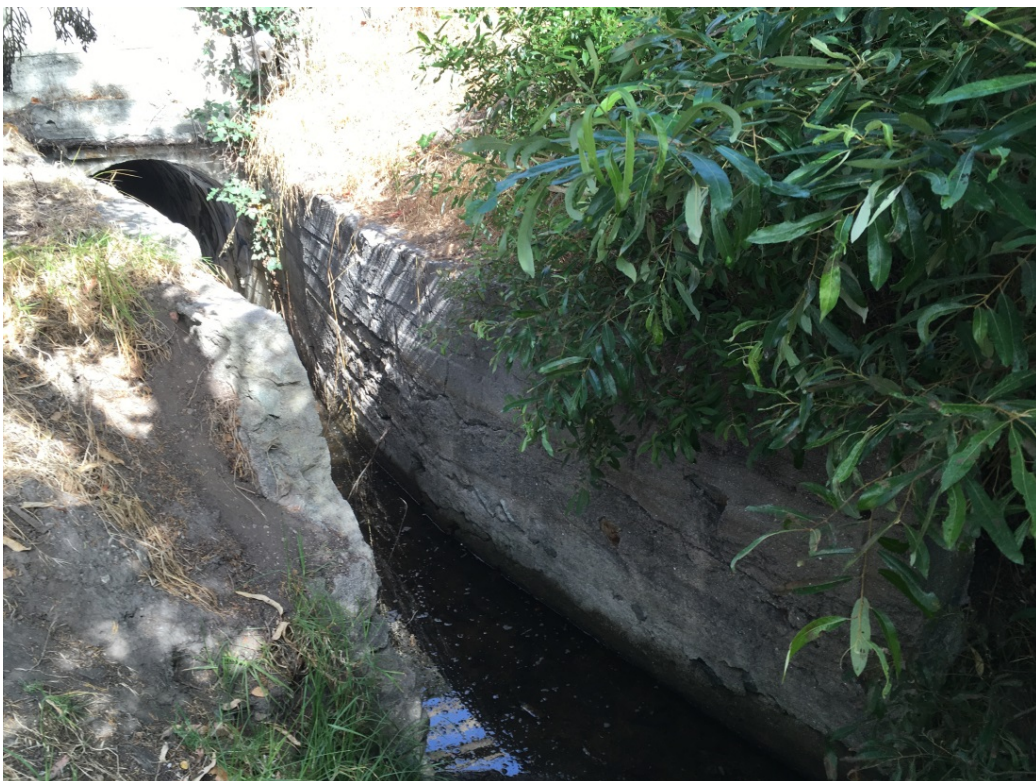
Site 5. Culvert outlet east of Pacific near library, facing structure. The outlet is armored for about 20 feet.
