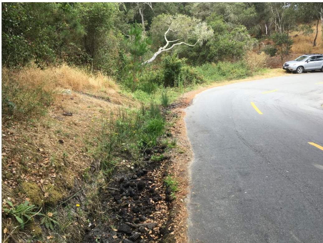
Site 21. Roadside ditch that catches seep water, looking west toward upstream reach of stream.
