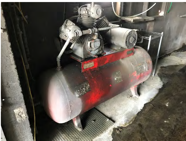
Photograph 5. Air compressor within carwash.
