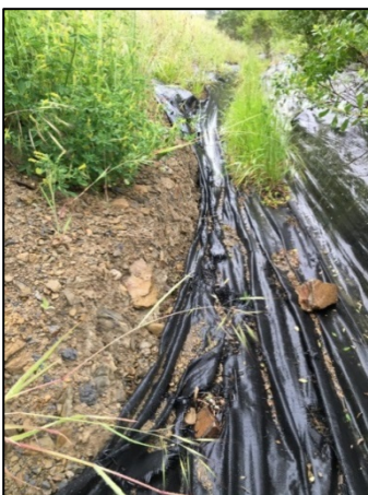
Photo 1: Northern Swale draining the watershed to the north of the central ridge in the Study Area. The swale is lined with a black tarp, which is disintegrating at places.
