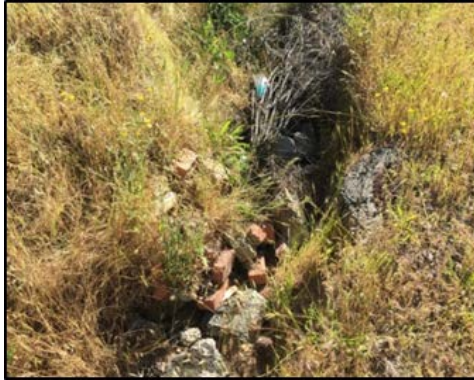
Photo 3: The downslope section of the roadside ditch. Ongoing erosion is transforming this ditch to a gully. This ditch is constructed entirely in uplands, does not drain wetlands, and is not connected to a tributary.
