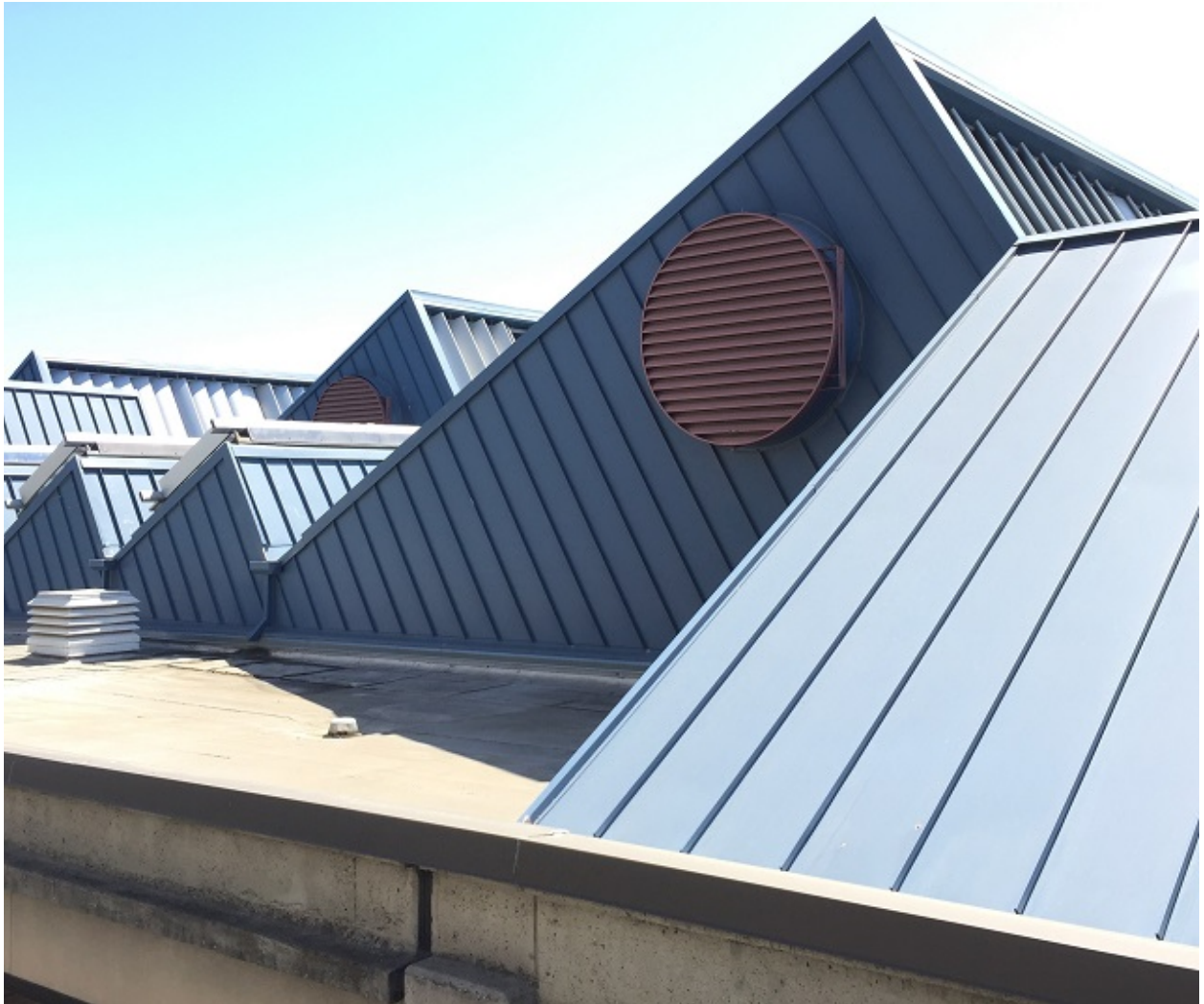
Figure 10. Bateson Building, Rooftop Sawtooth Monitors (ICF International 2015)
